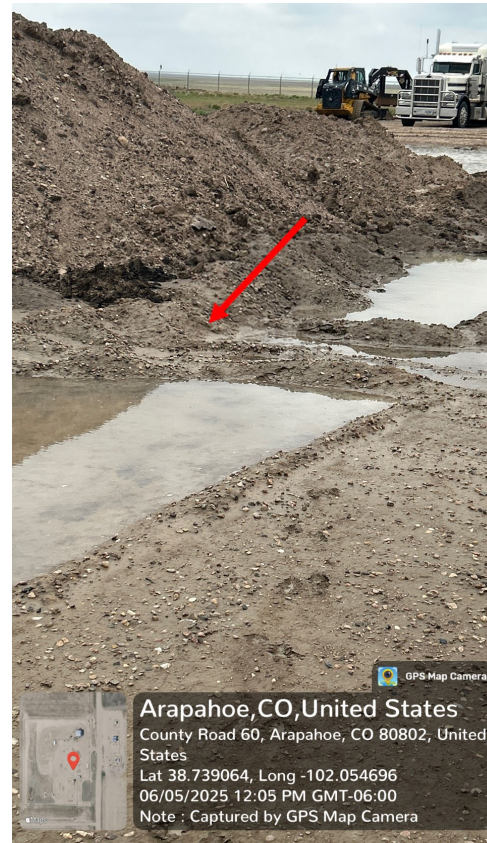
Photo 6 – Inadequate earthen berms
