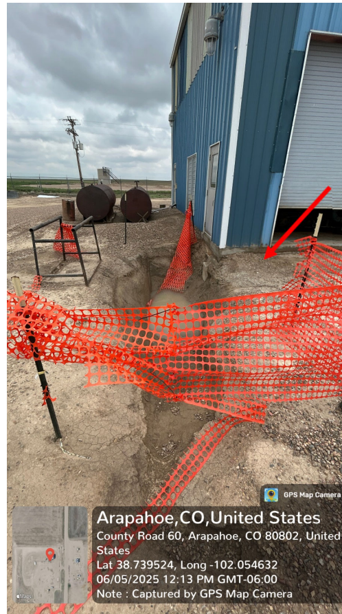
Photo 9 – Inadequate fencing
