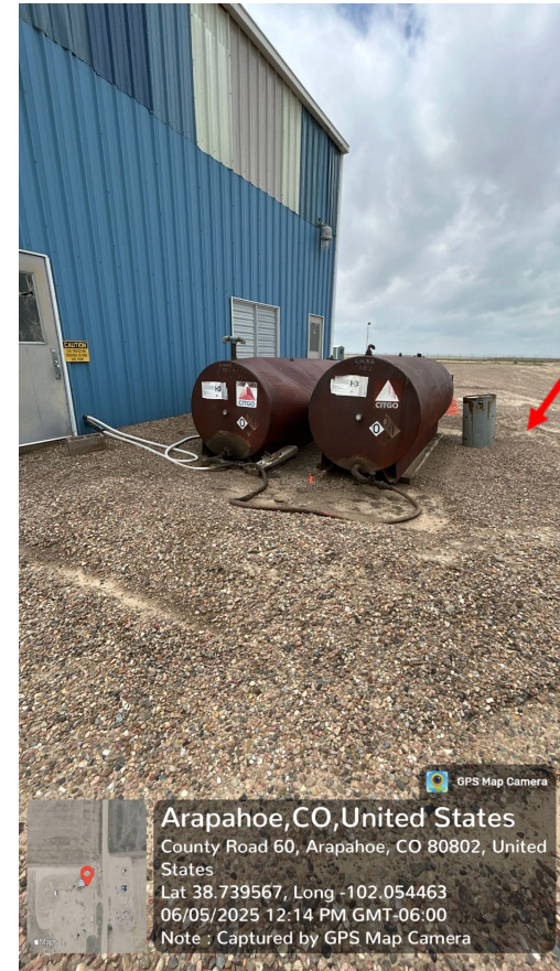
Photo 4 – Inadequate Berming
