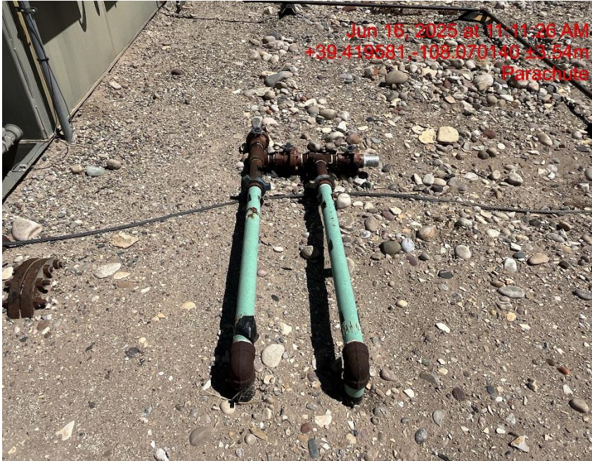
Photo # 8543 Multiple unused flowlines do not comply with CECMC 600 & 1100 series rules
