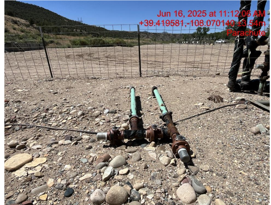
Photo # 8545 Multiple unused flowlines do not comply with CECMC 600 & 1100 series rules
