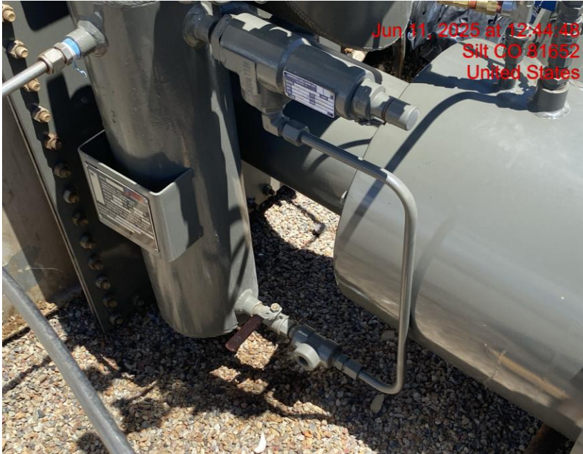
PRV Terminates in Unsafe Manner – Photo #09303
