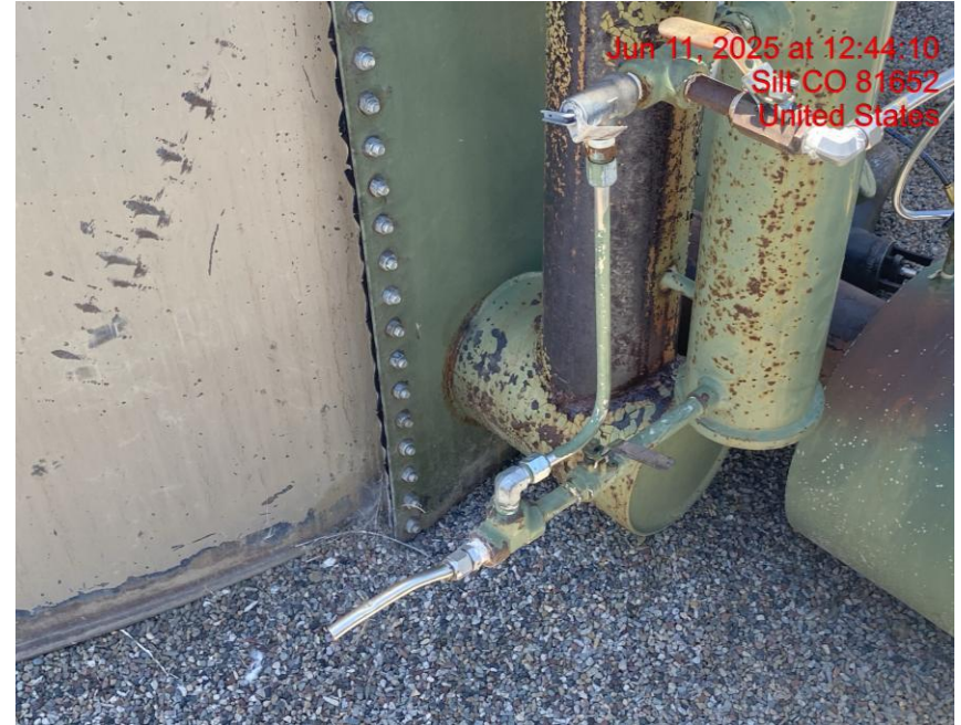
PRV Terminates in Unsafe Manner – Photo #09302
