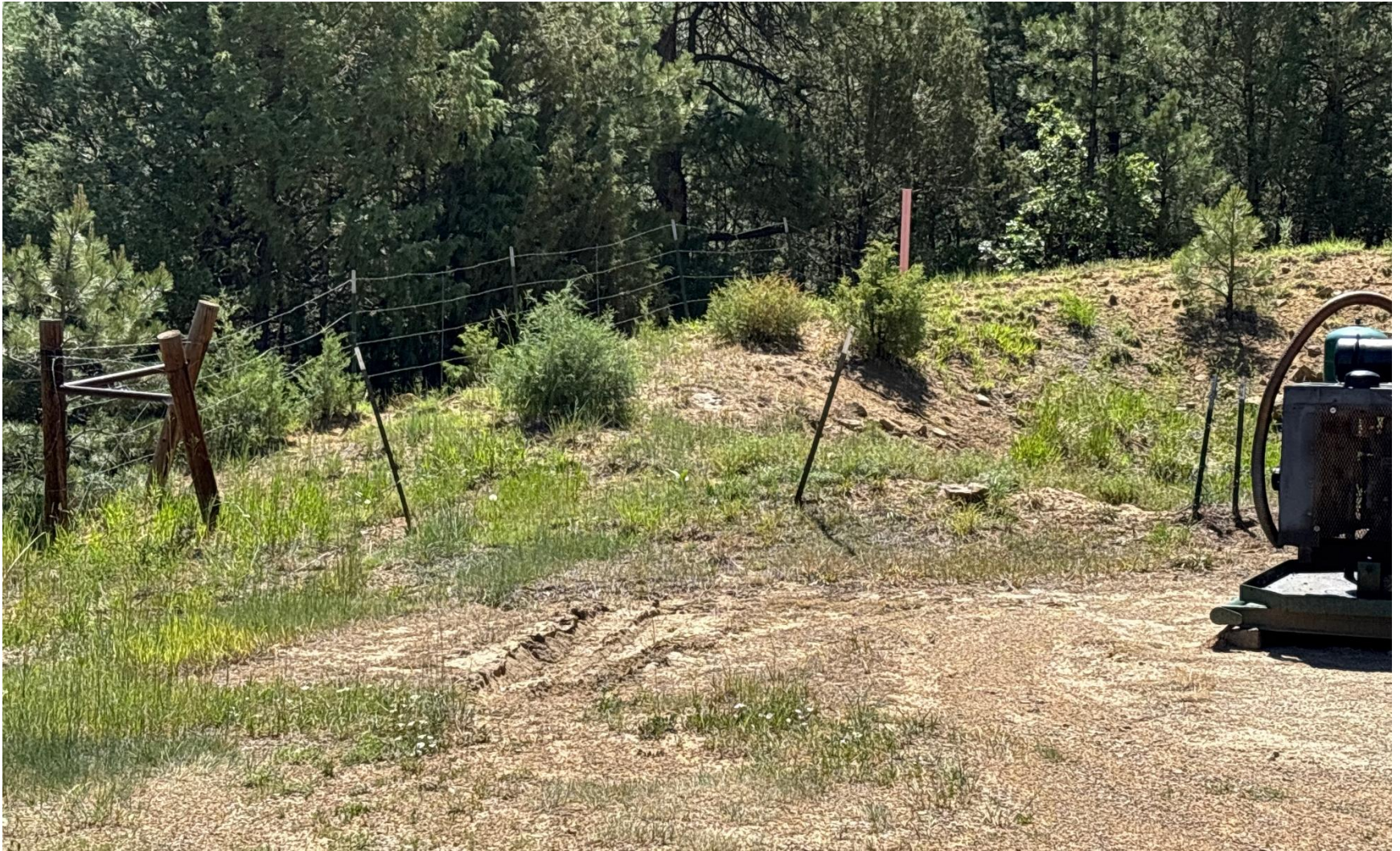
PHOTO 10: PART OF THE WIRES HAVE BEEN REMOVED FROM FENCE. REPAIR FENCE PER 1002 SERIES RULES. CA DATE 6-25-2025.
