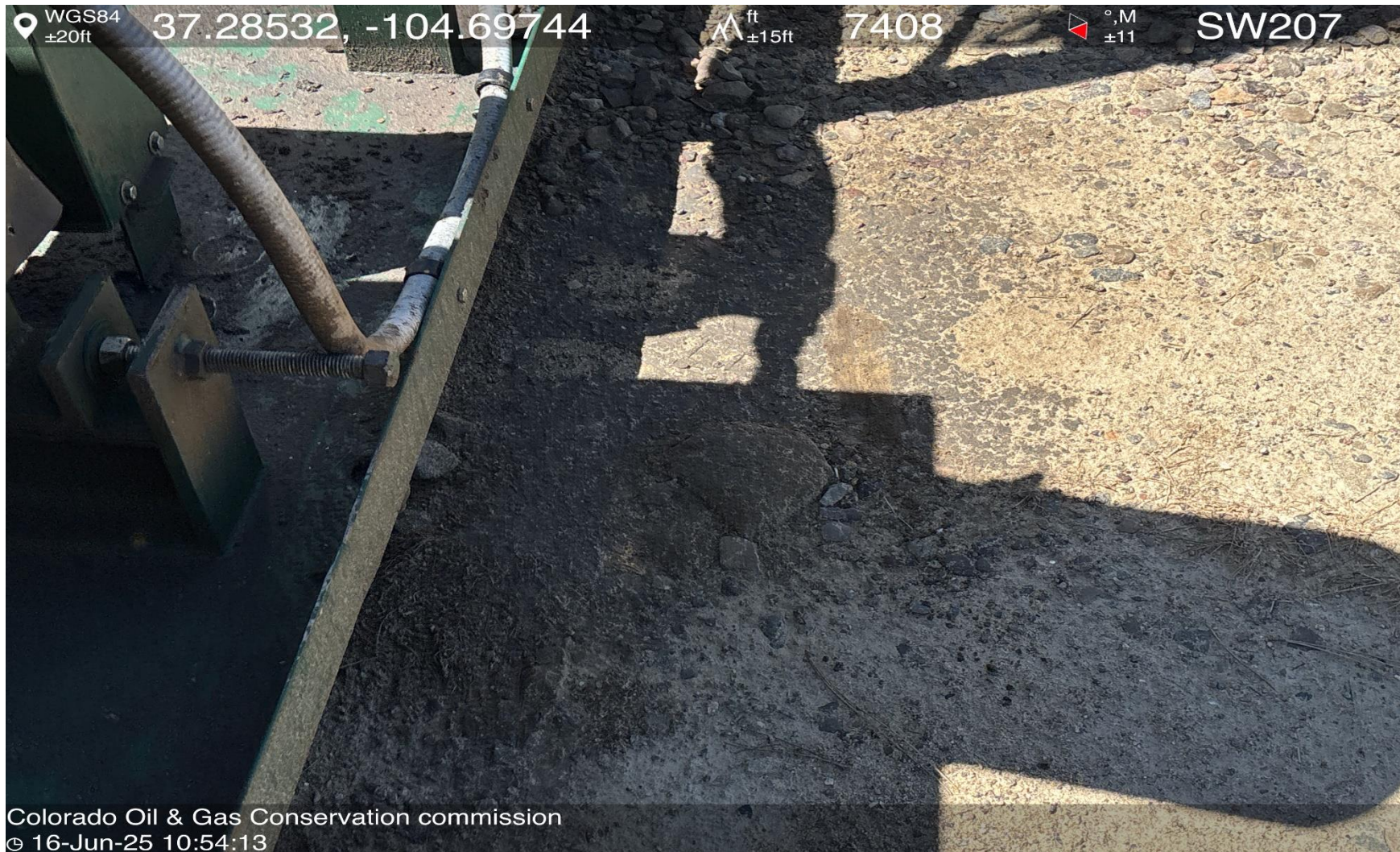
PHOTO 9: AREA OF IMPACTED SOIL AROUND COMPRESSOR SKID. Conduct maintenance on equipment, cleanup stained material and review self inspection processes. COMPLY WITH RULE 1002,(2).D. CA DATE 6-25-2025.
