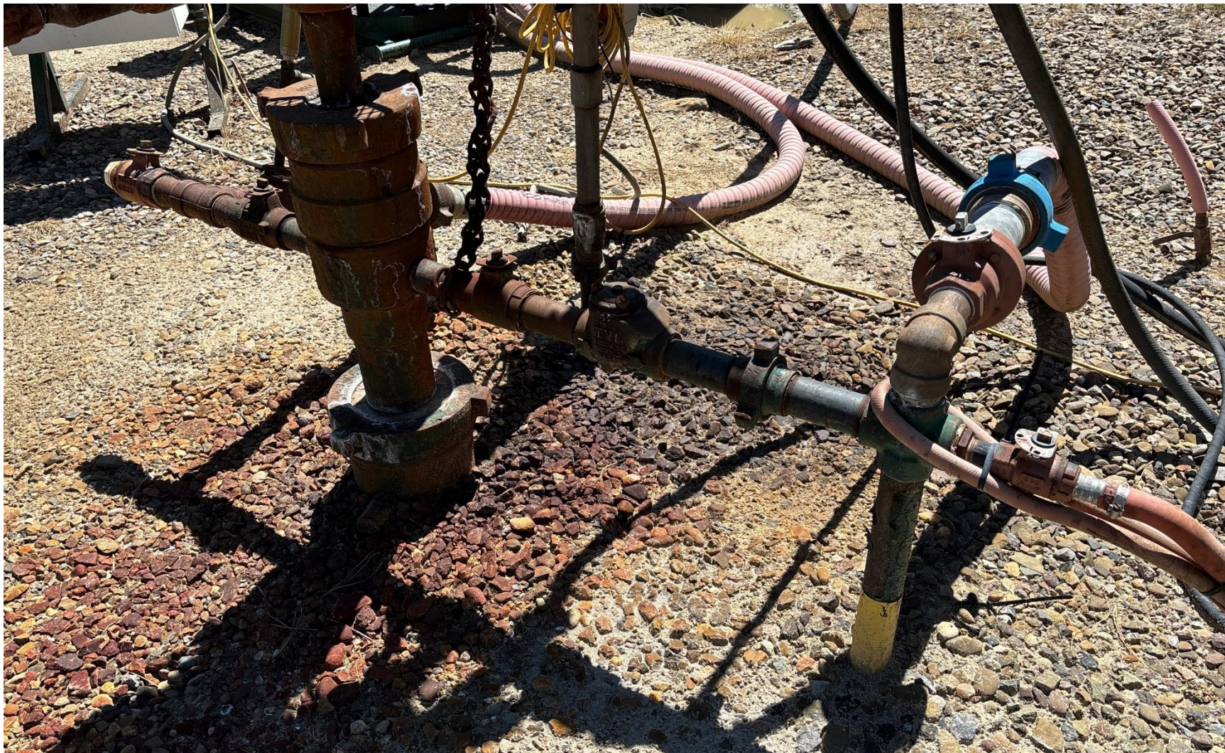
PHOTO 6: AREA OF IMPACTED SOIL AROUND WELLHEAD APPEARS TO BE FROM LEAKING DRIVEHEAD MOTOR SHOWN IN NEXT PHOTO. Conduct maintenance on equipment, cleanup stained material and review self inspection processes. COMPLY WITH RULE 1002,.(2).D. CA DATE 6-25-2025.
