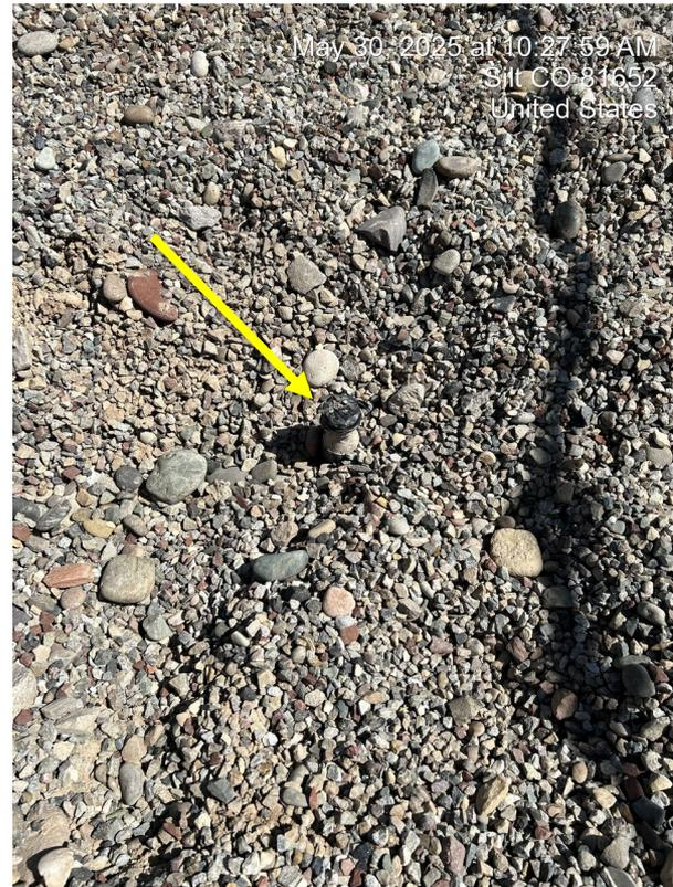
**Photo 3:** Photo taken from between the separator equipment on the west end of the Location. Photos shows riser associated with abandoned wells/equipment remaining on the Location. The riser requires cutting, capping and removal.
