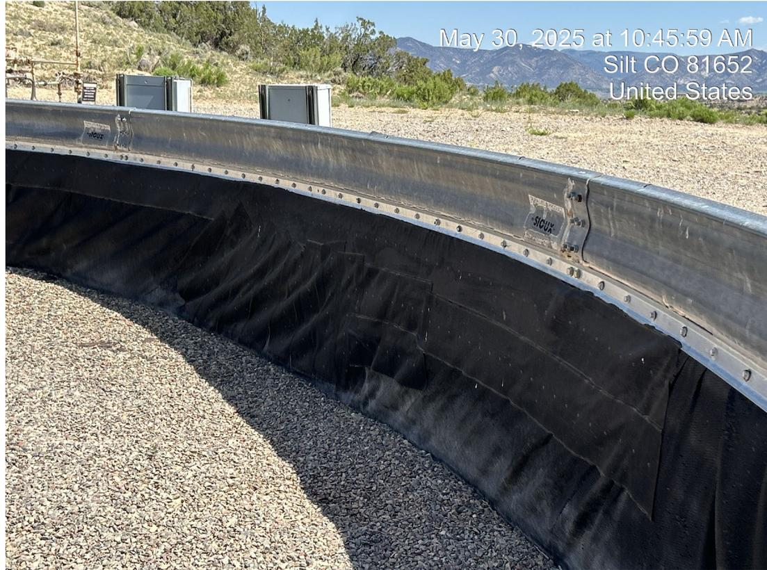
**Photo 6:** The tank battery liner appears to be aging and may need replaced soon.
