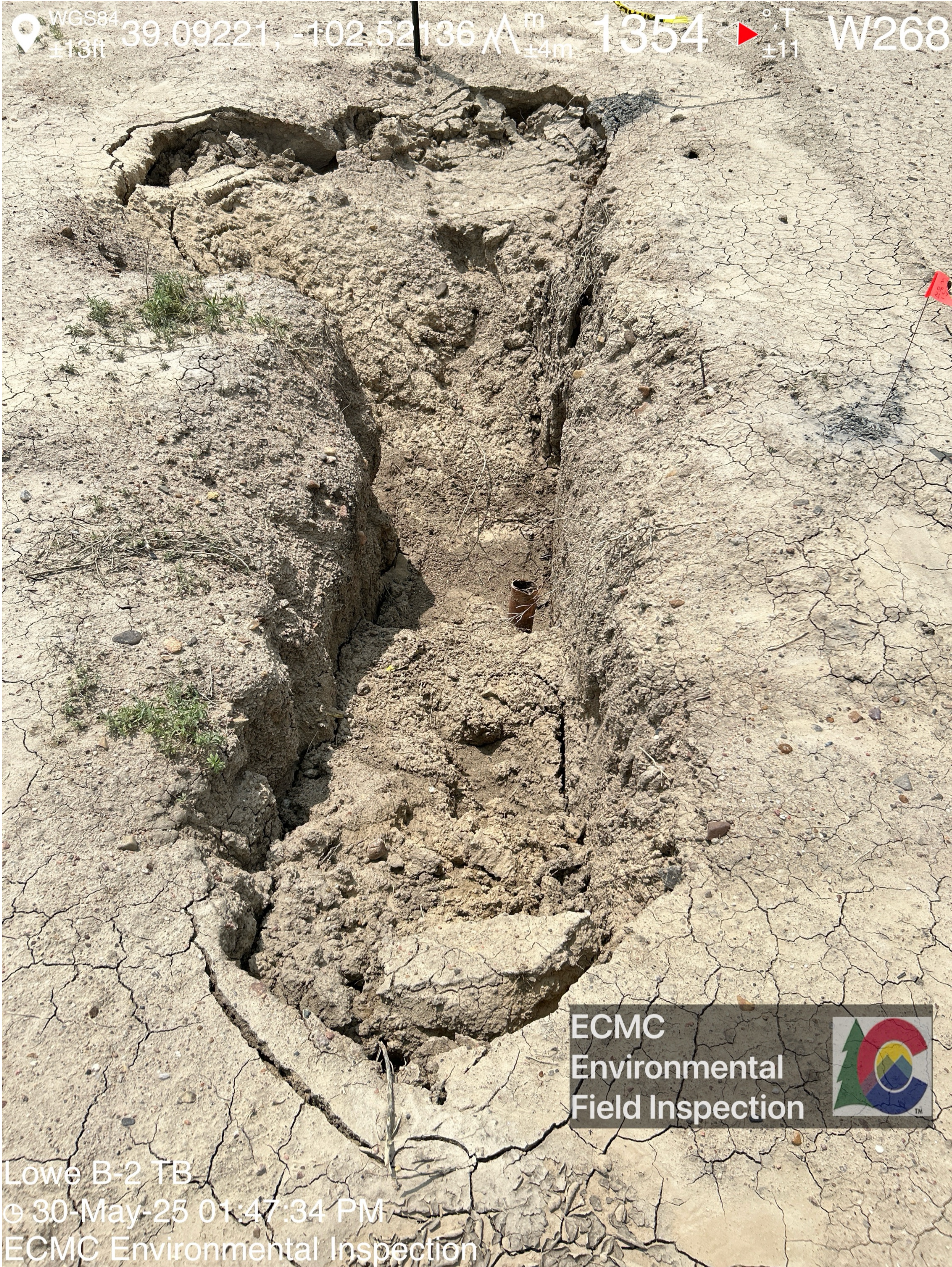
An uncapped riser is visible within one of the trenches/excavations.
