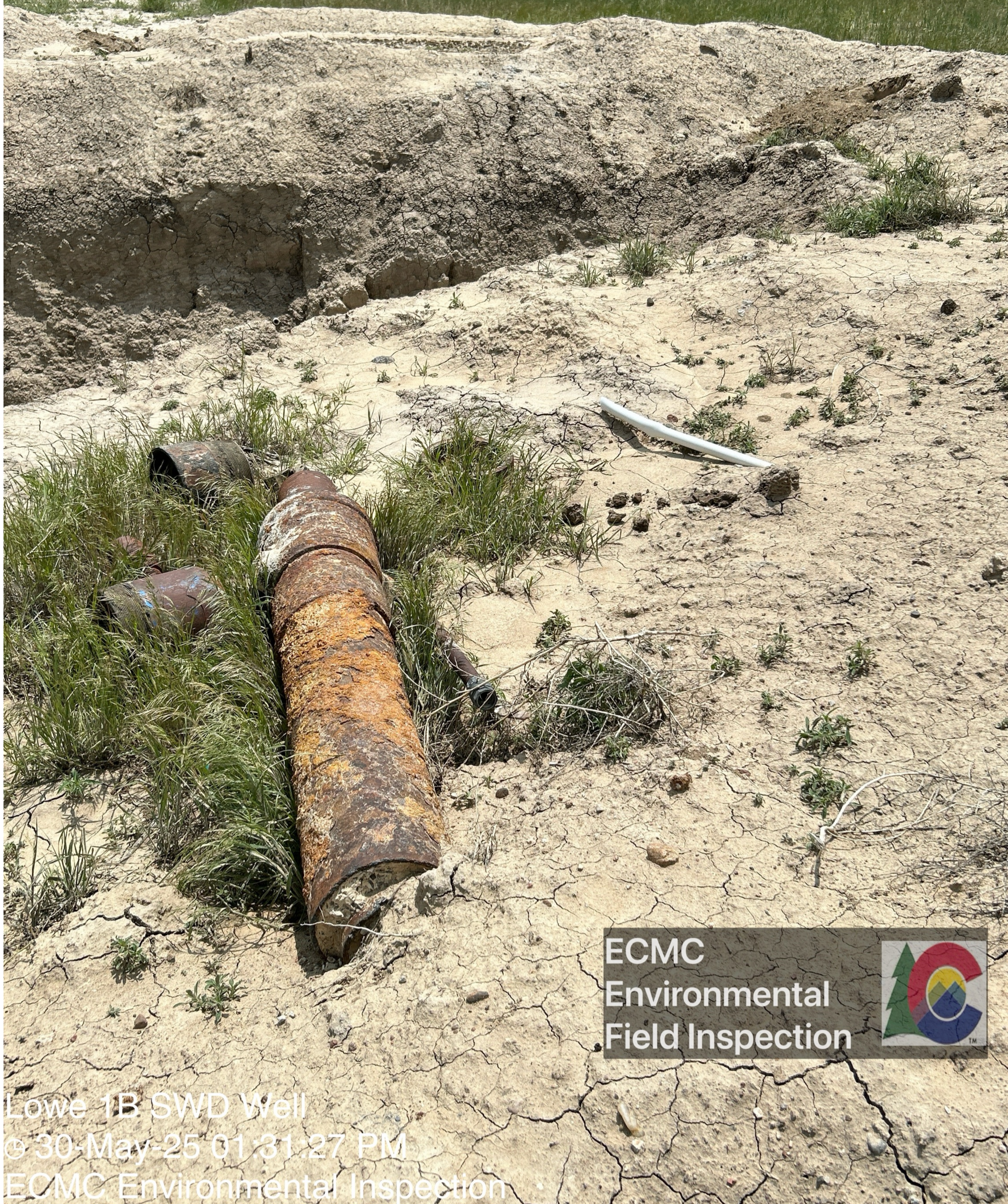
The well casing and a segment of white plastic pipe are visible adjacent to the wellhead excavation.
