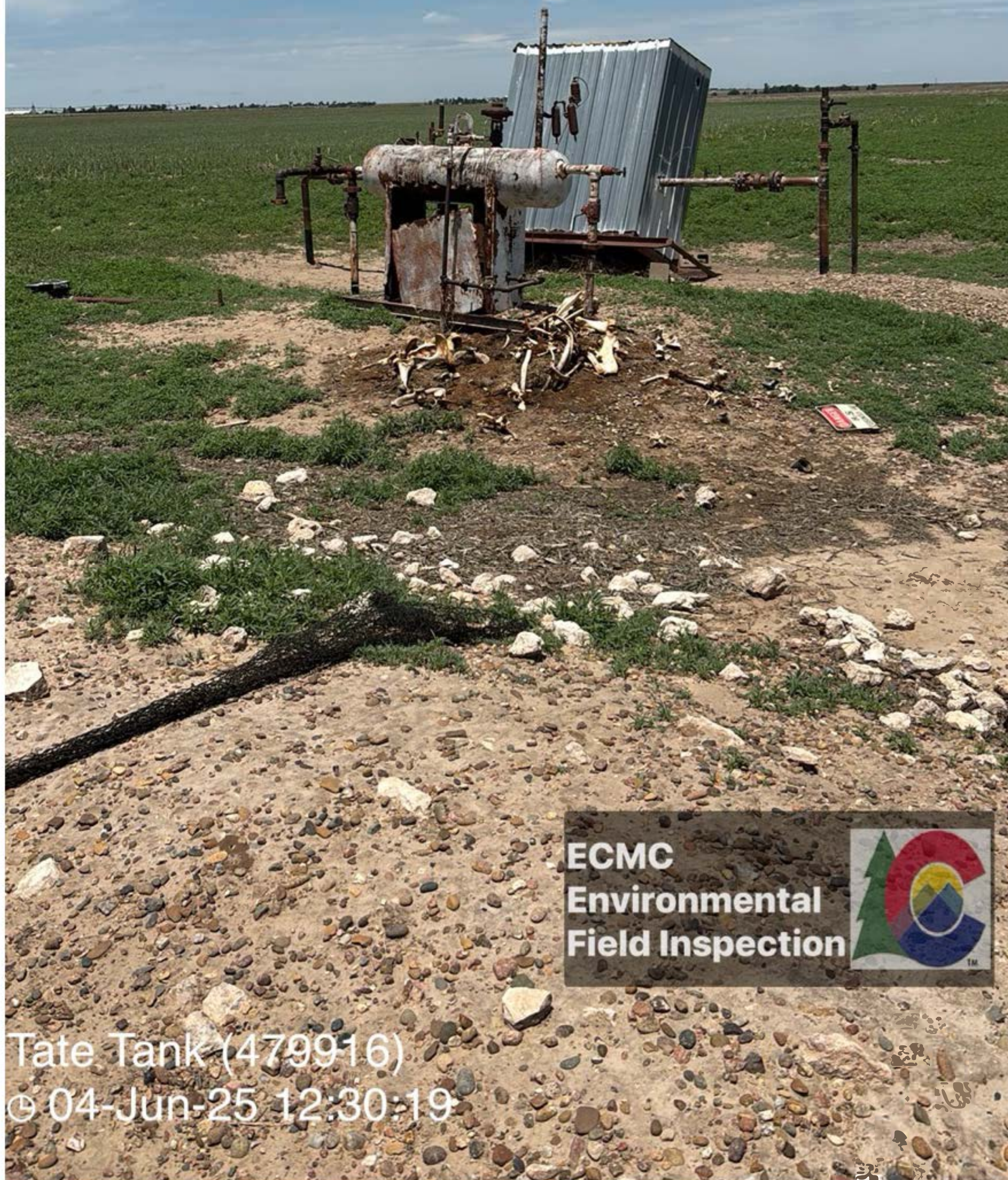
Cattle carcass, trash/debris - torn wildlife protection equipment (netting), weeds, fallen signage.
