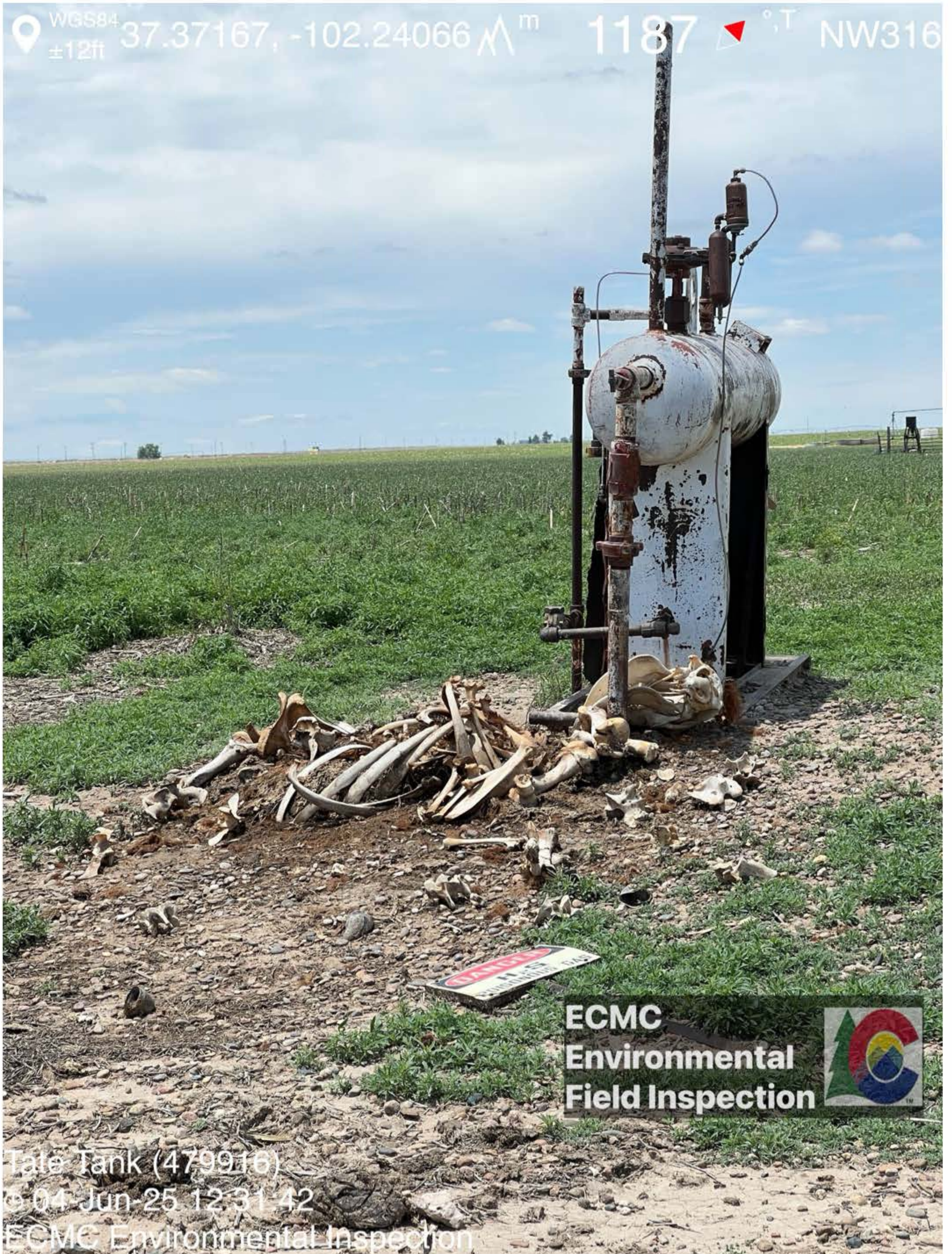
Cattle carcass adjacent to separator and piping, trash/ debris - torn wildlife protection equipment (netting), weeds, fallen signage.
