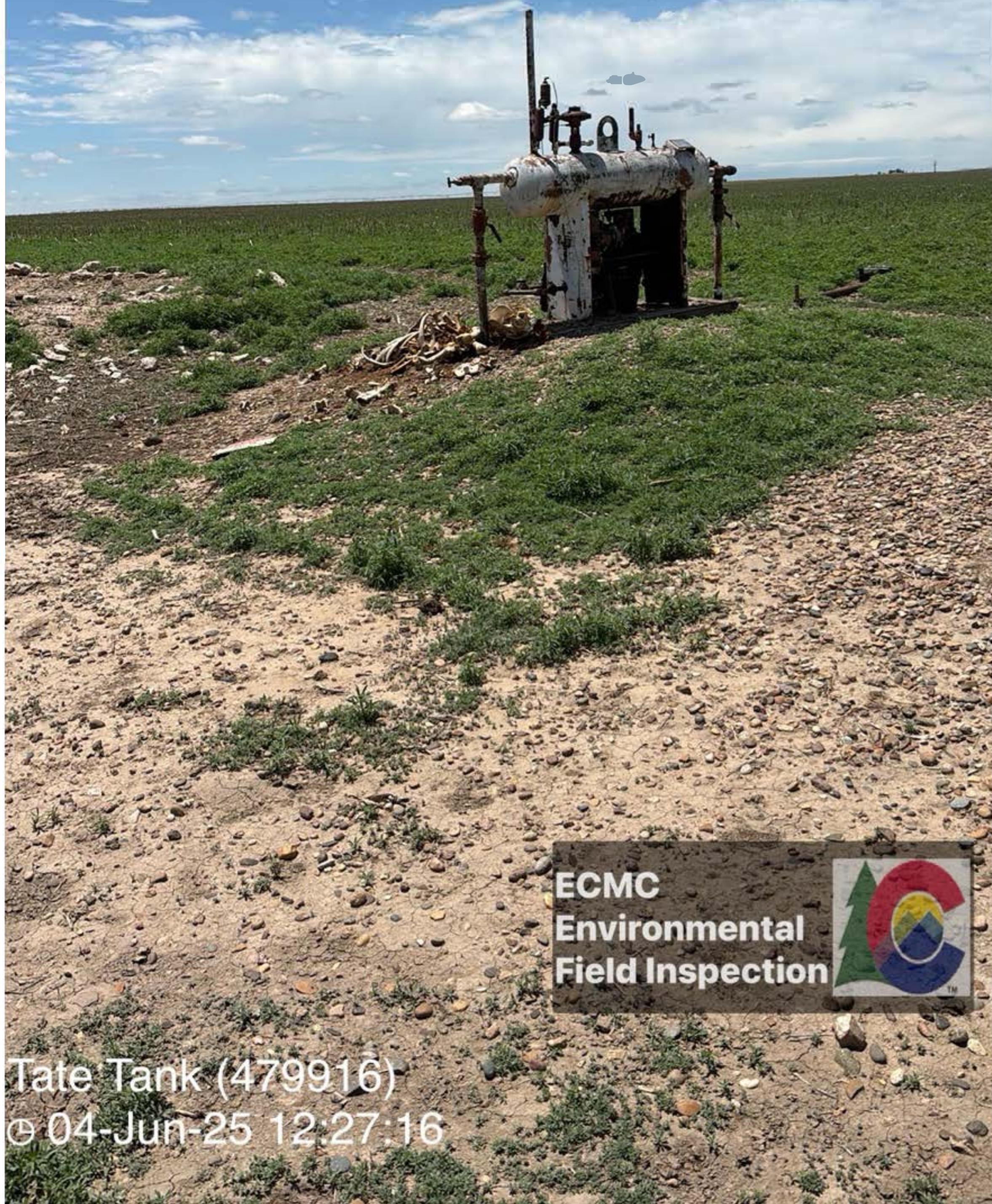
Cattle carcass, weeds, fallen/inadequate signage at separator.
