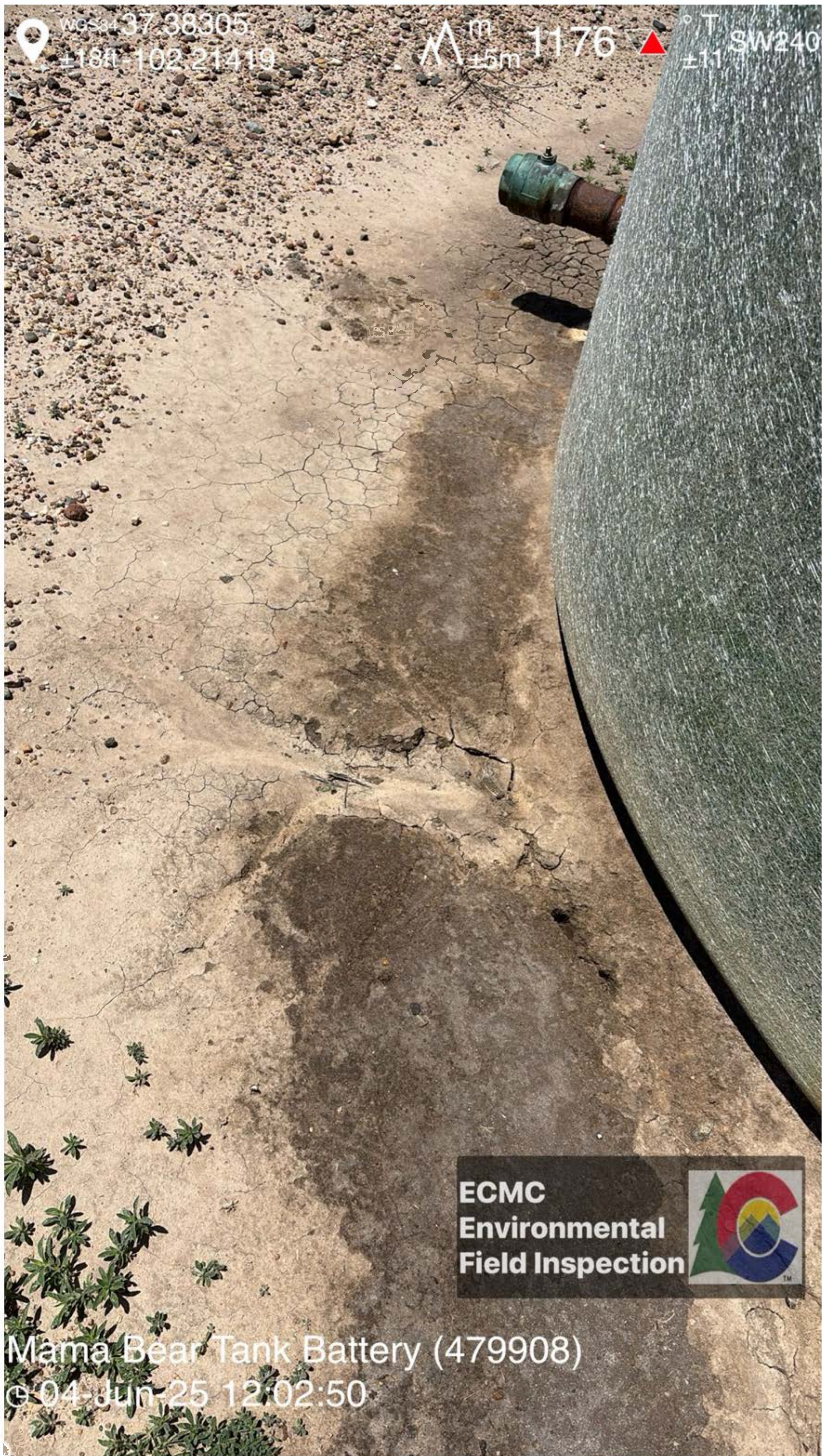
-Stained soil observed around the base of the 100-bbl open-top fiberglass produced water storage tank -Weeds
