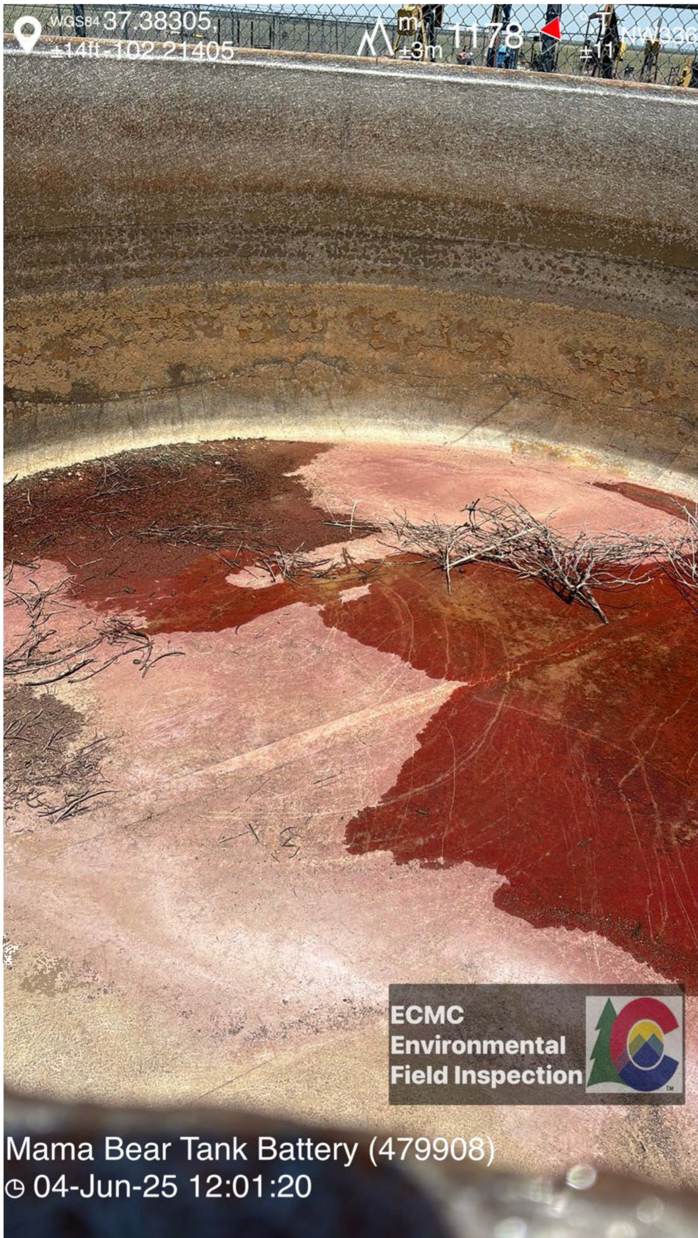
-Wildlife protection equipment (netting) is missing on the 210-bbl open top fiberglass produced water storage tank (empty at time of inspection)
