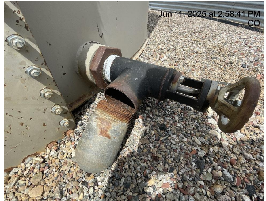
Photo # 8321 Open ended load line
