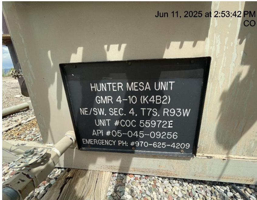
Photo # 8322 Emergency phone # on sign at separators incorrect/# is disconnected & not in service/not in compliance with CECMC rules.
