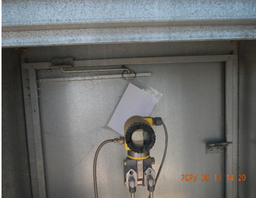
3. Gas Meter inside Meter Box.
