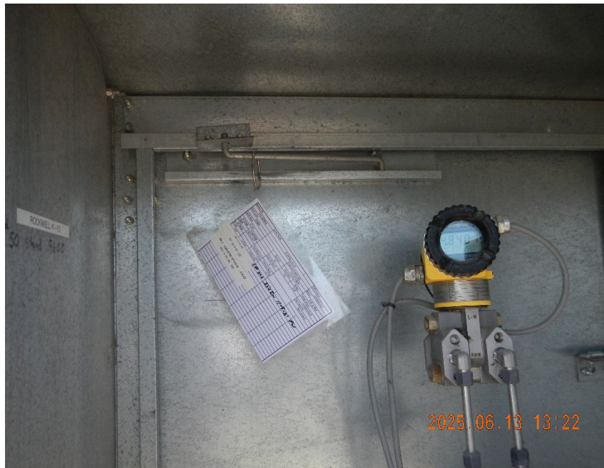
3. Gas Meter inside Meter Box.
