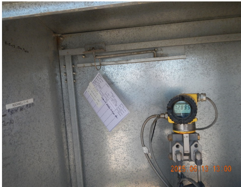
3. Gas Meter inside Meter Box.
