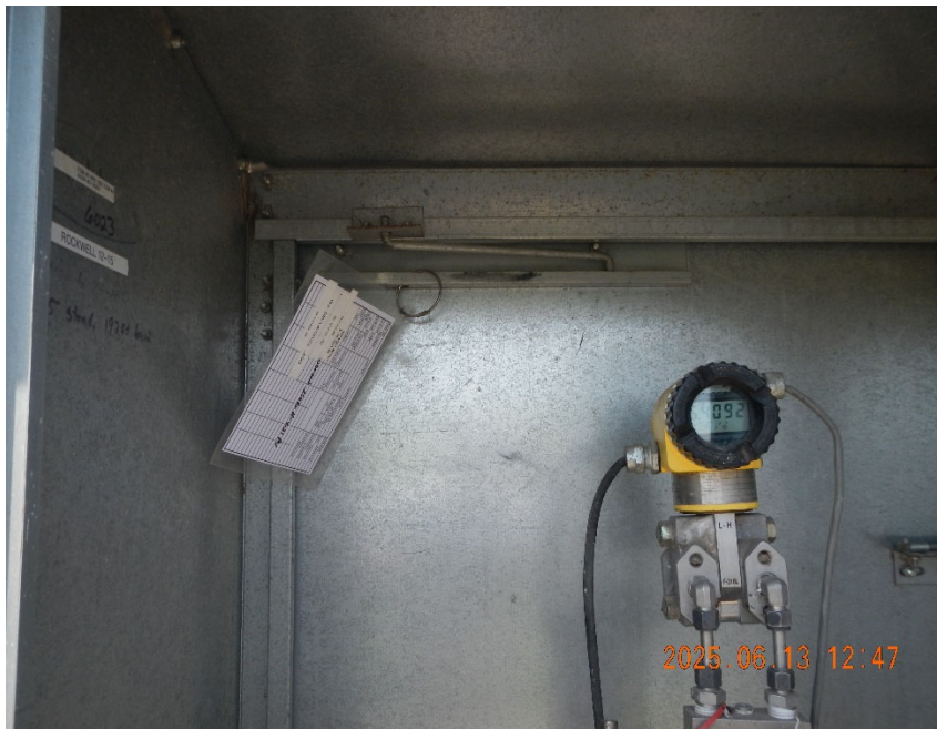
5. Gas Meter inside Meter Box.
