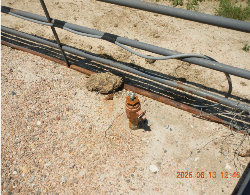
3. Flowline riser with valve and plug at wellhead.
