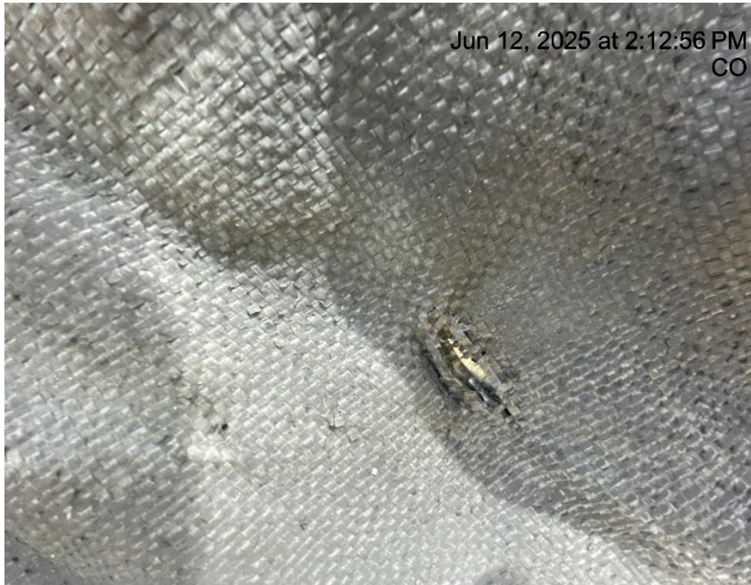
Photo # 8640 Hole in liner/liner needs maintenance
