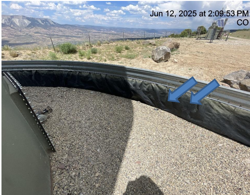
Photo # 8632 Holes in liner/liner needs maintenance
