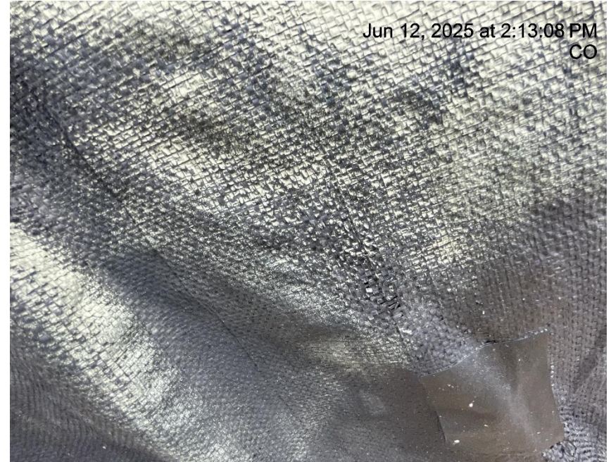
Photo # 8645 Liner deteriorating/liner needs maintenance
