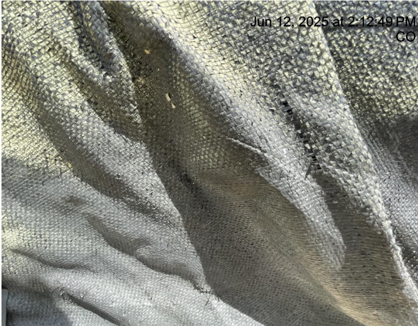
Photo # 8642 Liner deteriorating/liner needs maintenance
