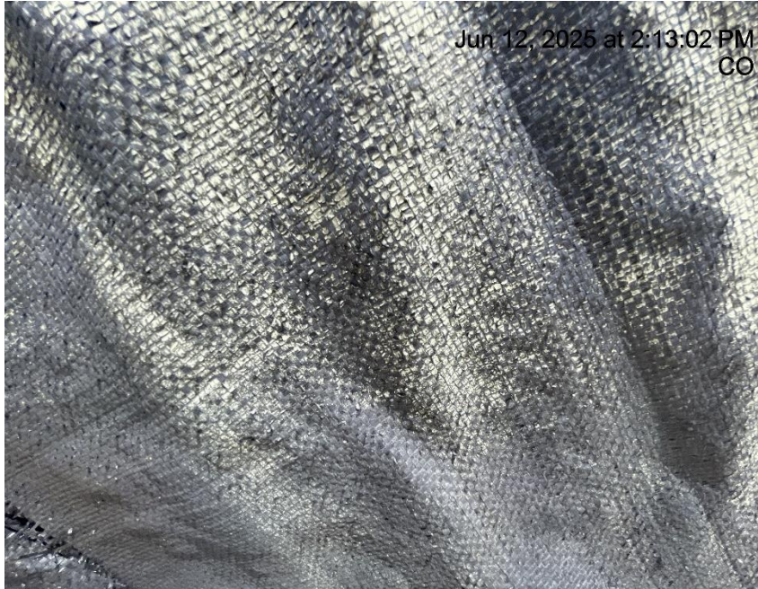
Photo # 8644 Liner deteriorating/liner needs maintenance
