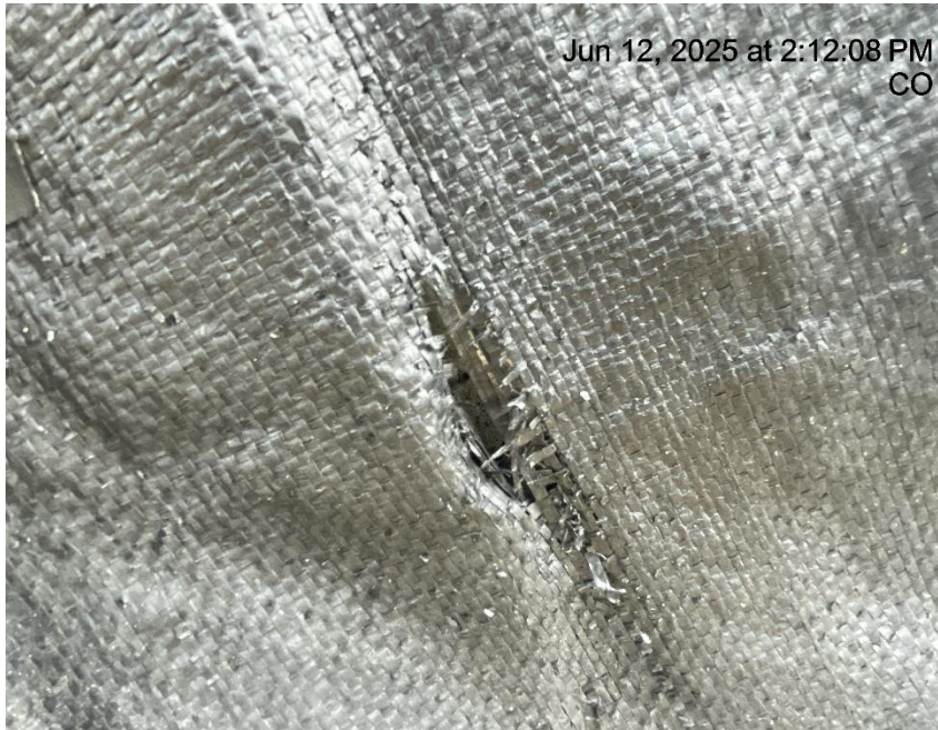
Photo # 8638 Hole in liner/liner needs maintenance
