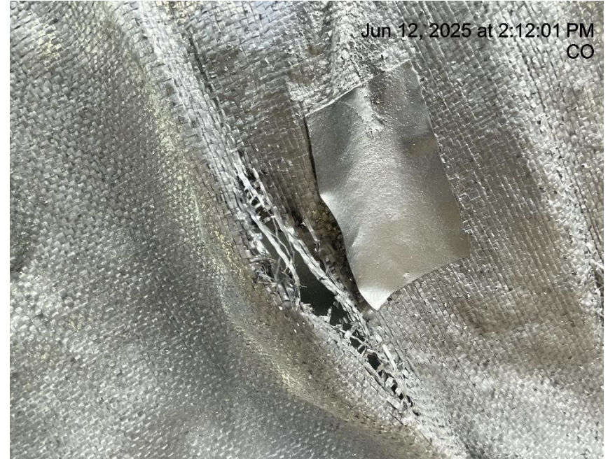
Photo # 8637 Hole in liner/liner needs maintenance
