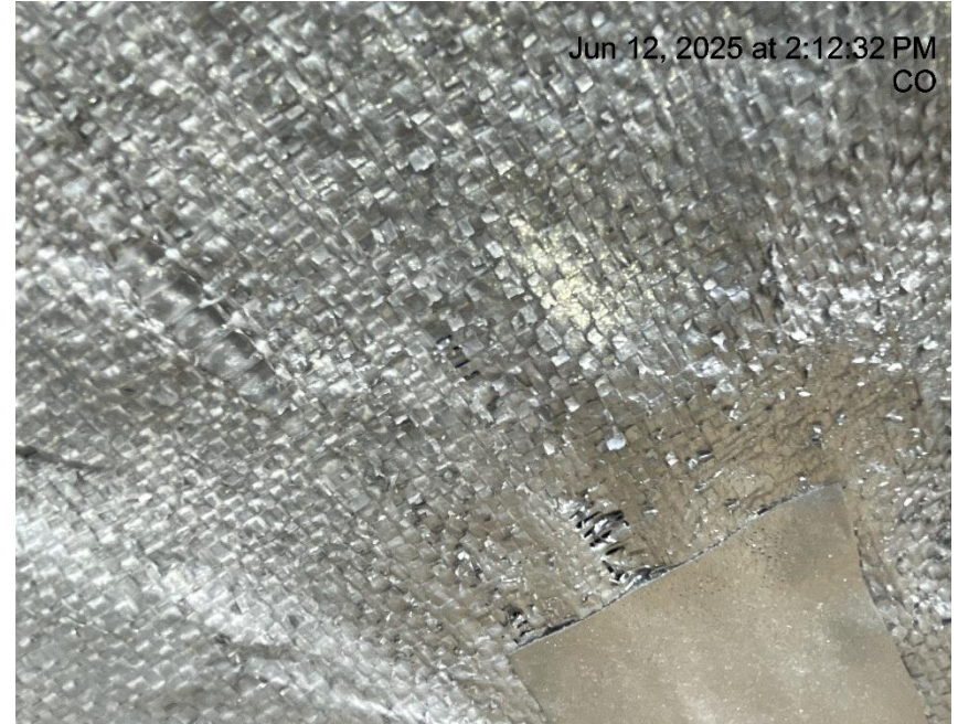
Photo # 8643 Liner deteriorating/liner needs maintenance
