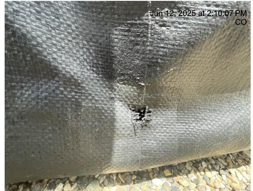
Photo # 8635 Hole in liner/liner needs maintenance
