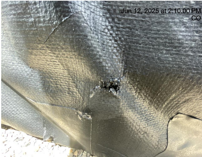
Photo # 8634 Hole in liner/liner needs maintenance
