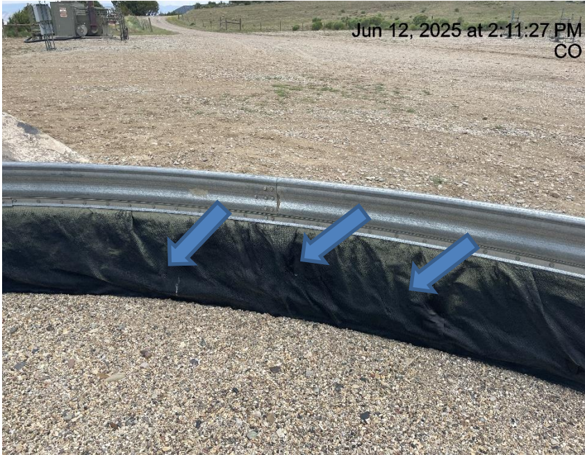
Photo # 8636 Holes in liner/liner needs maintenance
