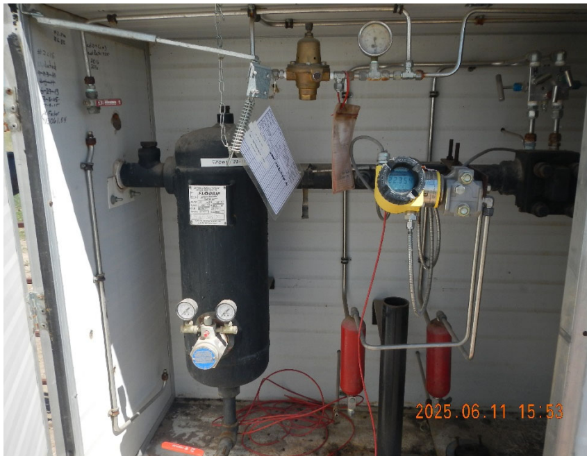
3. Dehydrator and Gas Meter inside Meter Box.
