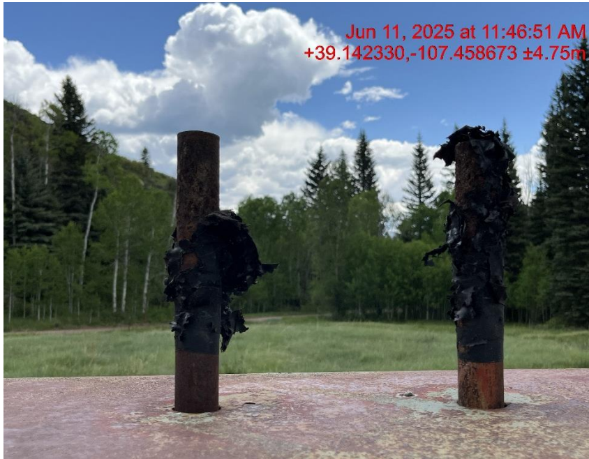
Photo # 8271 PRV vent line & Rupture disc vent line does not comply with CECMC pressure safety device rules
