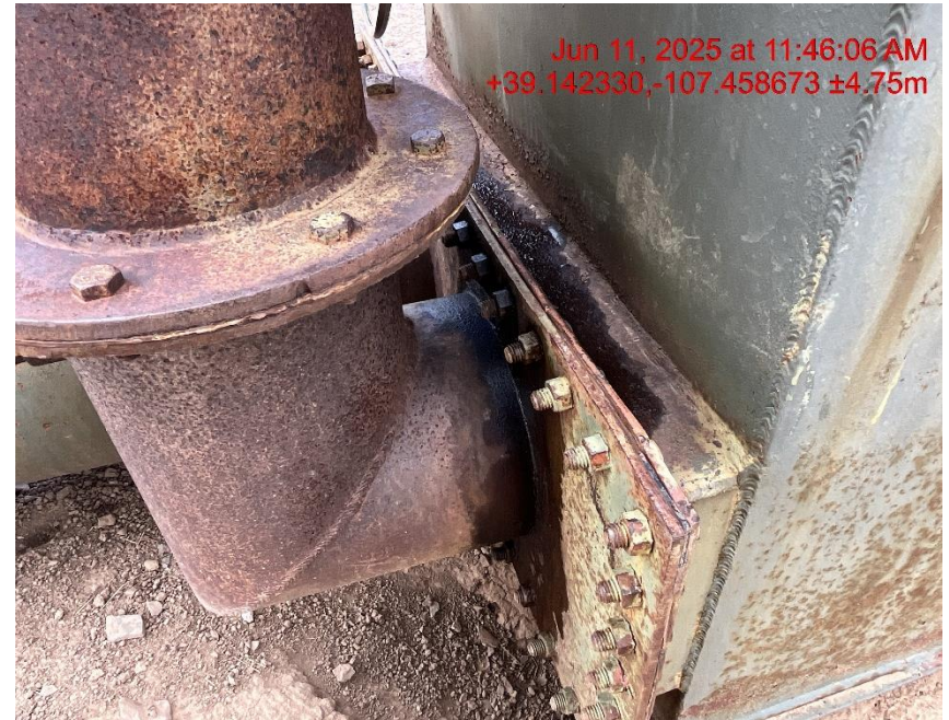
Photo # 8268 Staining around heater on separator
