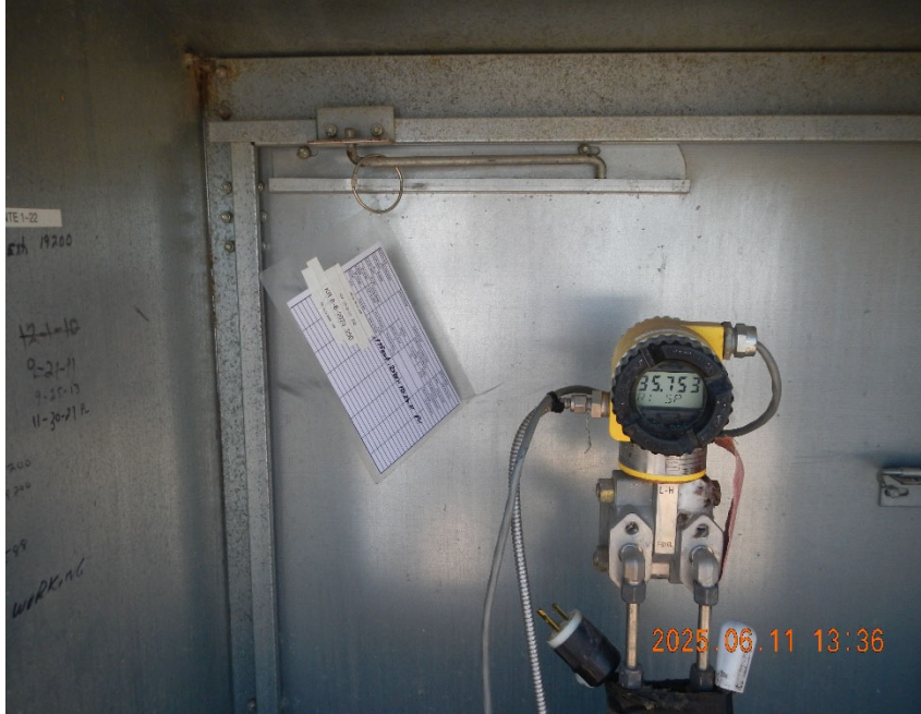
3. Gas Meter inside Meter Box.
