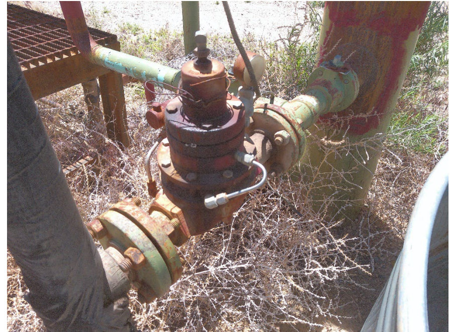
Valve with audible gas leak.
