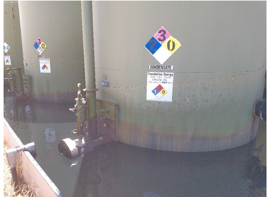
Produce Water/Condensate fluid level inside berms.
