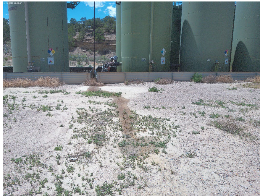
Spill area from leaking berms.
