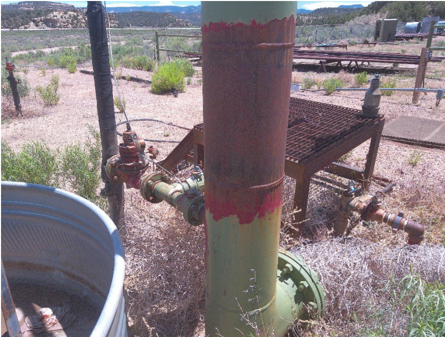
Flowline riser with audible gas leak
