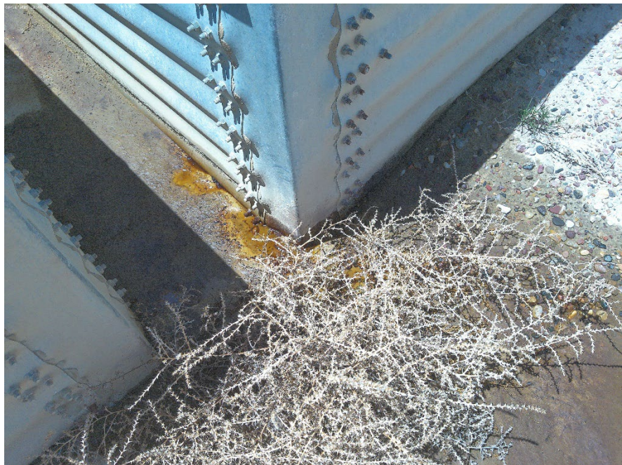
Leaking berm liner on SE corner of tank berms
