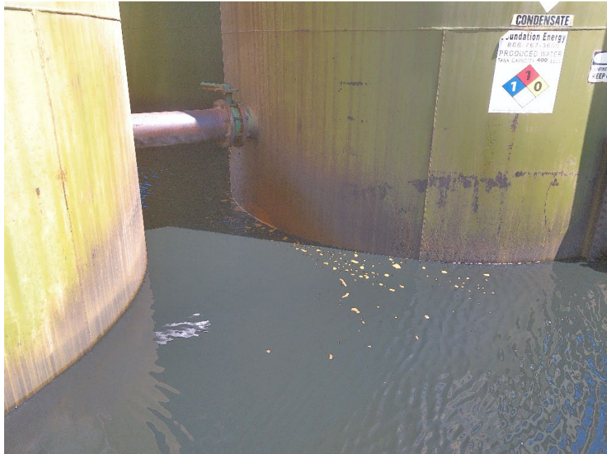
Leaking valve on Produced Water/ Condensate tank
