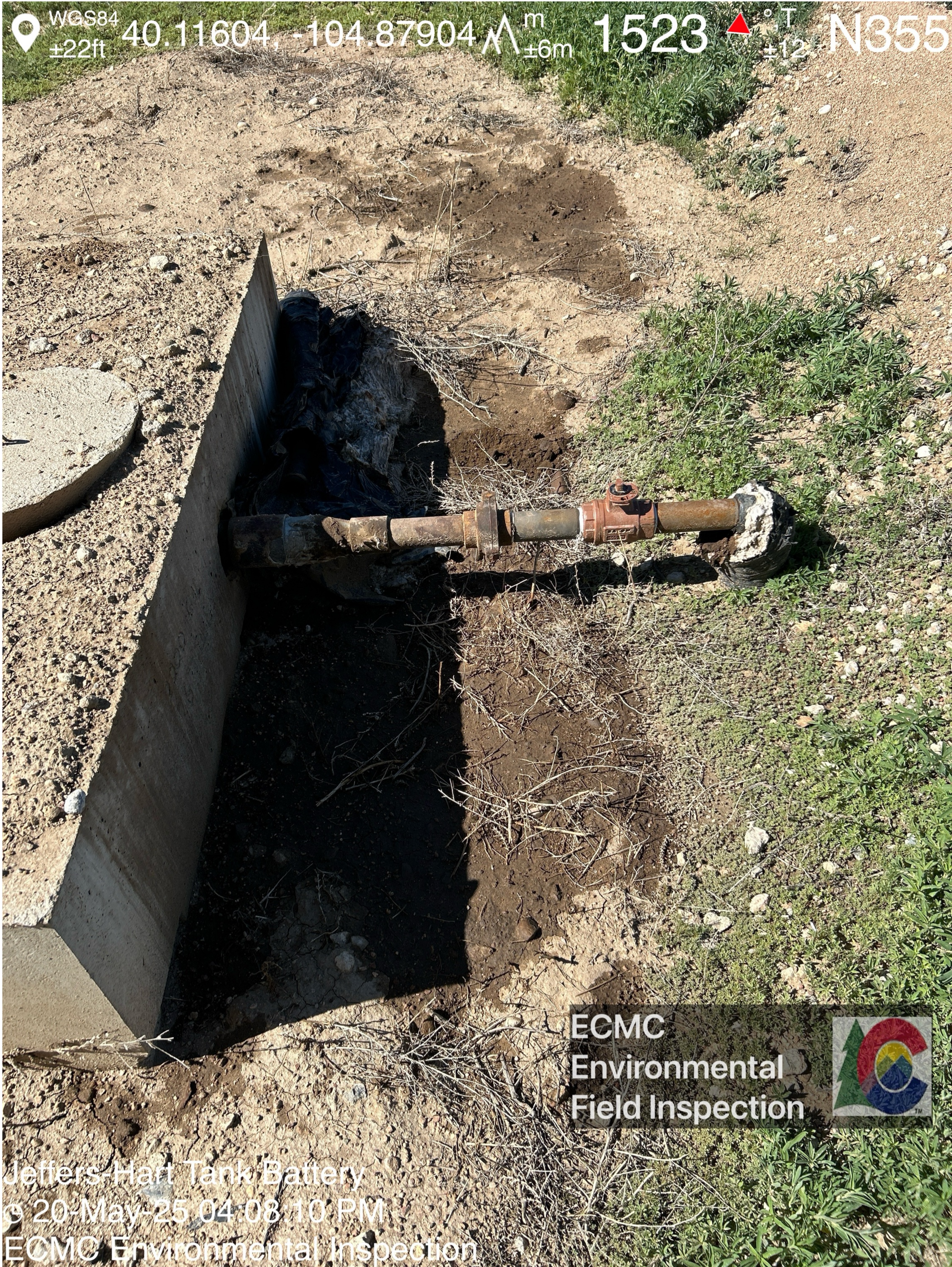
Insulation appears to have been removed from the produced water dump line and lies adjacent to the vessel (trash). Patches of stained soil are visible adjacent to the produced water vessel. A petroleum hydrocarbon odor was observed when the stained soil was disturbed.
