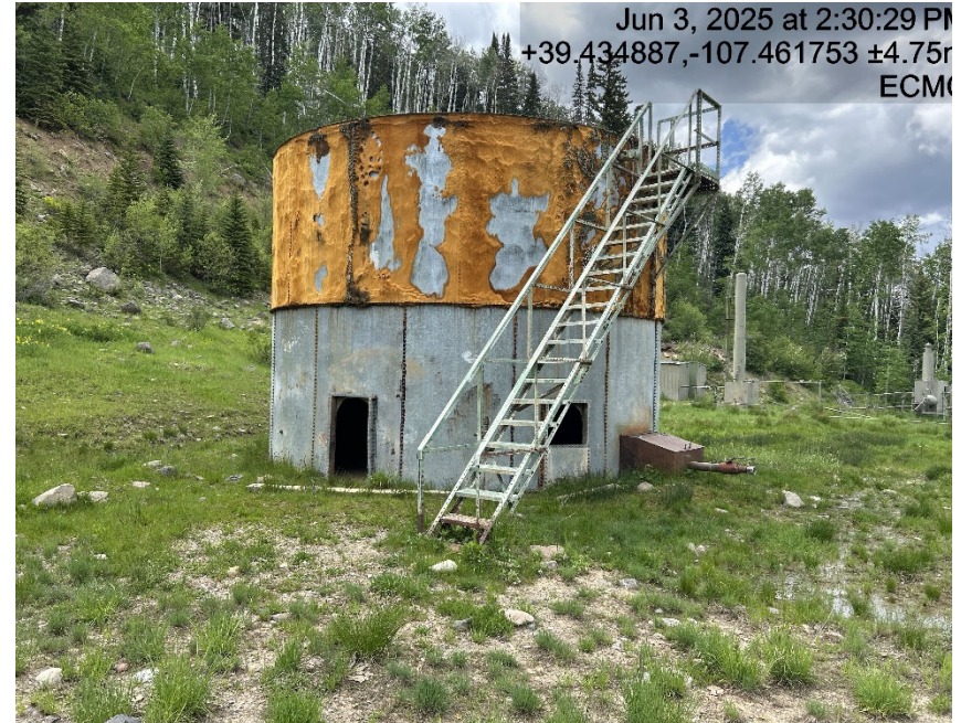
Unknown tank/ no secondary containment/ open holes for wildlife to enter/ no battery signage/ unused equipment/ weeds
