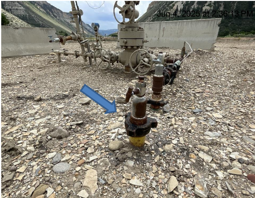
Photo # 6391 Unused flowline does not comply with CECMC rules
