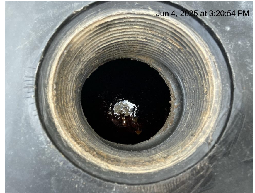
Photo # 6556 Failure to maintain chemical BMP – Chemical tank containment approximately 3/4 full of fluid/BMP insufficient to contain possible spill
