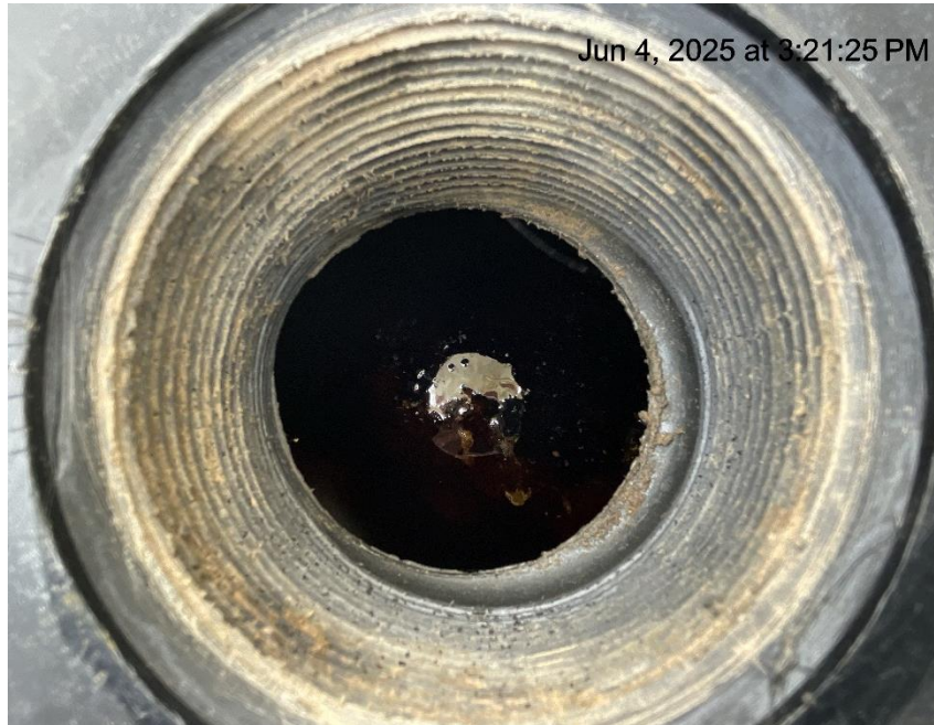
Photo # 6555 Failure to maintain chemical BMP - Chemical tank containment approximately 3/4 full of fluid/BMP insufficient to contain possible spill
