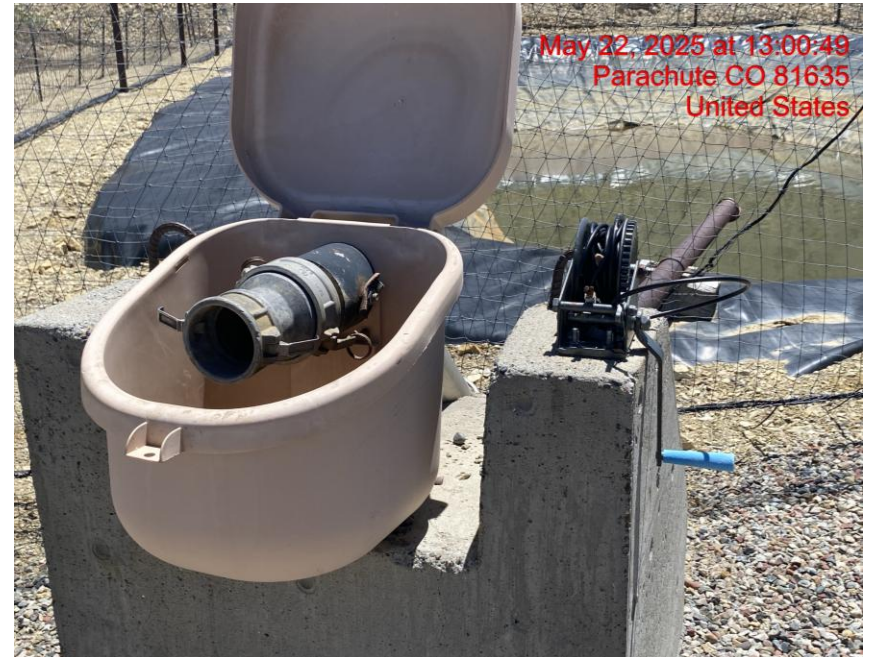
Open-Ended Line Into Pit – Photo #09081
