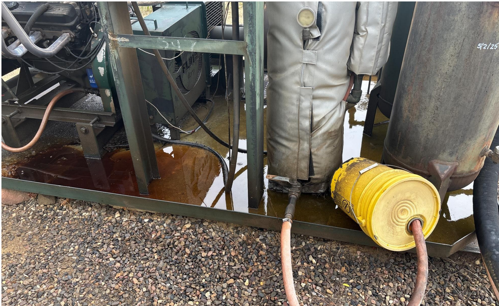
PHOTO 5: OILY WASTE IN COMPRESSOR SKID. DRAIN OILY WASTE REPAIR ALL LEAKS AND REMOVE IMPACTED SOIL PER RULE 1002..(2).D & 1002.f.(2)B, Comply with general provisions of the oil and gas act for wildlife protection AND SB-181. CA DATE 6/5/2025.
