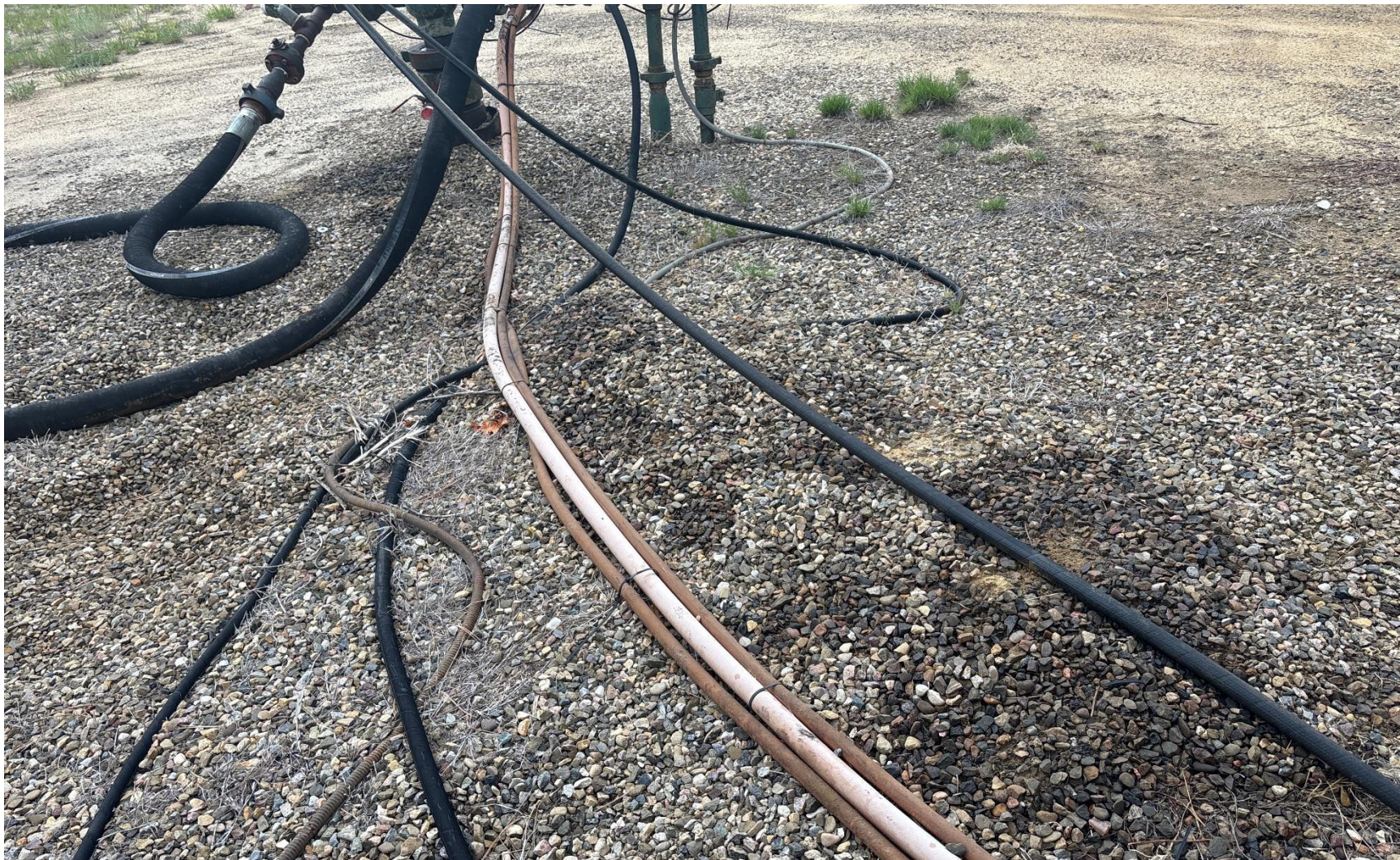
PHOTO 4: AREA OF IMPACTED SOIL/GRAVEL ALONG THE HYDRO. LINES FROM COMPRESSOR TO DRIVEHEAD. Conduct maintenance on equipment, cleanup stained material and review self inspection processes. COMPLY WITH RULE 1002,(2).D. CA DATE 6/15/2025.
