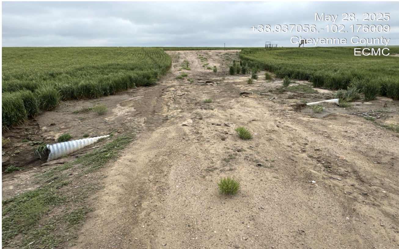
Photo 3. The culvert along the access road near the wellsite has washed out and needs to be repaired. Previous CA was not completed.
