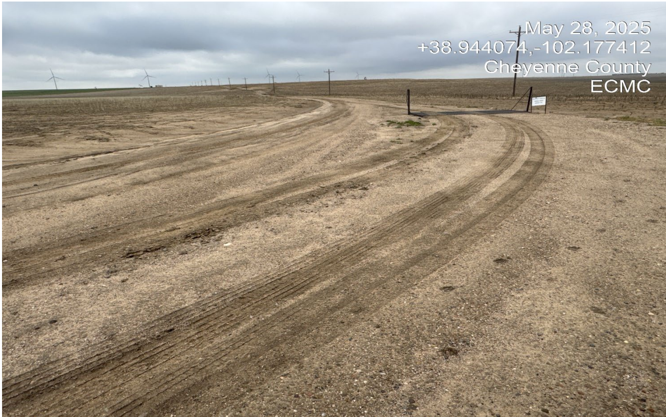
Photo 1. Facing southwest at the beginning of the access road. There is vehicle traffic going around the cattle guard causing widening of the road and unnecessary surface disturbance.
