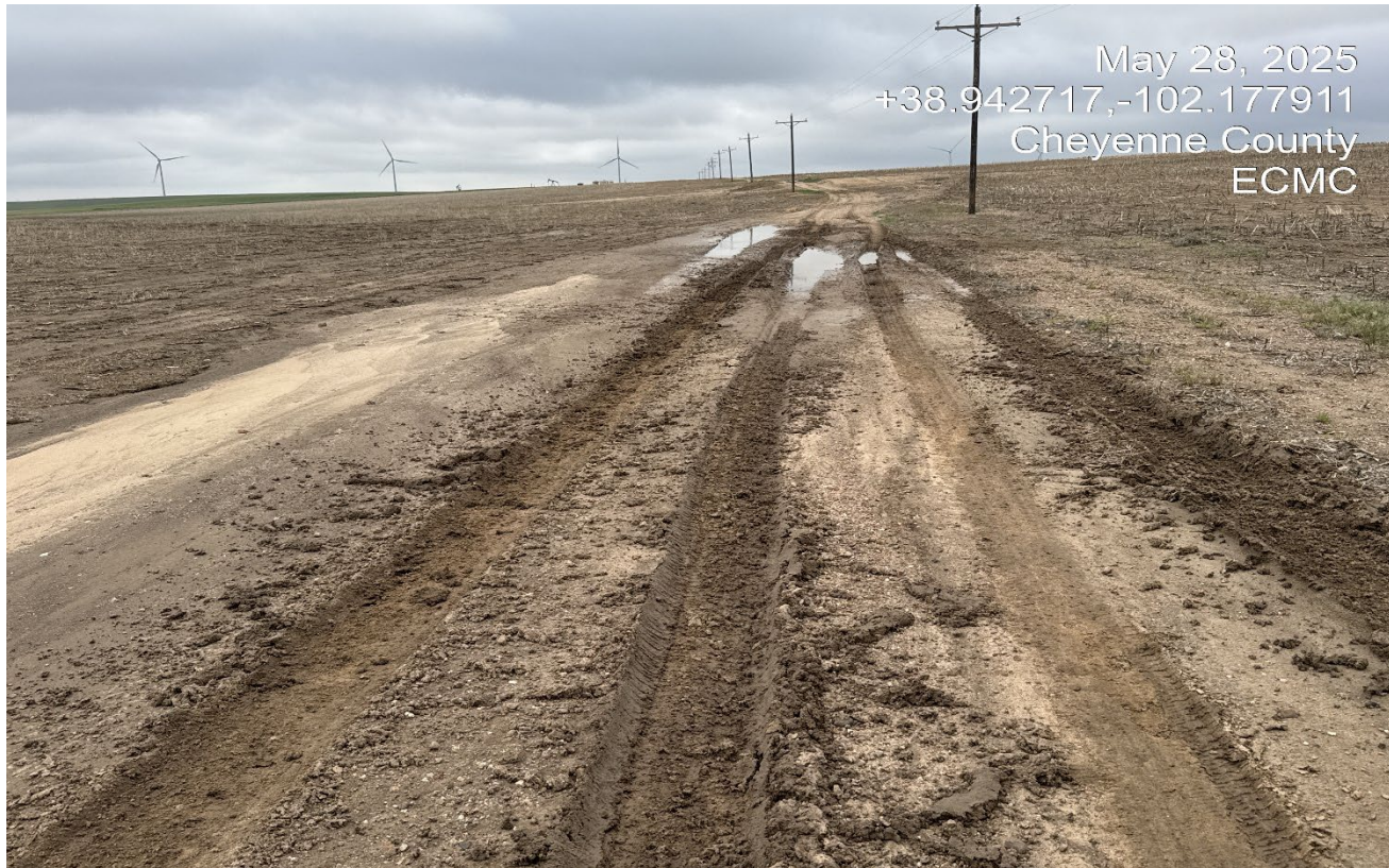
Photo 2. Facing south along the access road. The access road is rutted and not maintained in this area. Vehicle are widening the road at this area.
