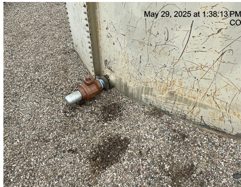
Photo # 4647 Staining in secondary containment
