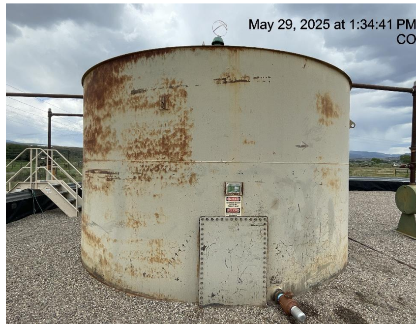
Photo # 4649 Production tank not in compliance with rule 425
