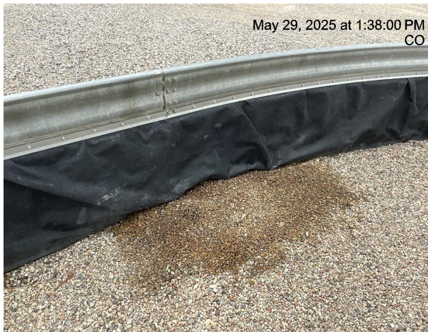
Photo # 4646 Staining in secondary containment
