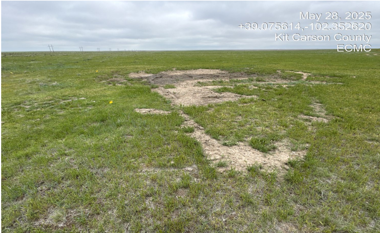
Photo 1. Facing north where pipe riser has been removed. Disturbance area will need to be reclaimed.
