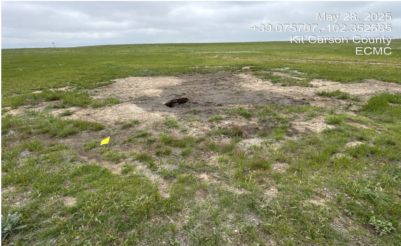
Photo 2. Facing east where associated pipe riser was removed. There is subsidence and topsoil will be need to regrade this area.
