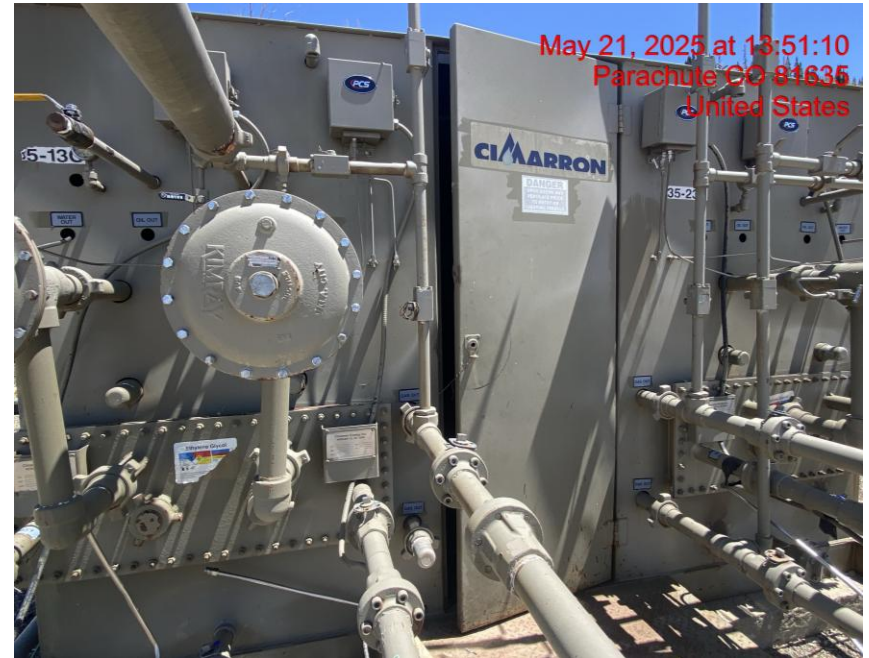
Open Door on Separator/Wildlife Entry Hazard – Photo #08956
