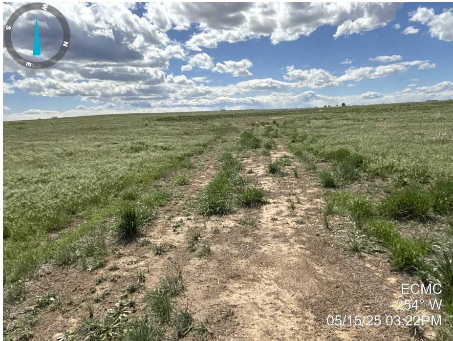
Photo 5. Photo taken from the access road, facing West towards the well location. Photo illustrates that final reclamation activities appear to have taken place, but vegetation has not established to Rule 1004 standards.
