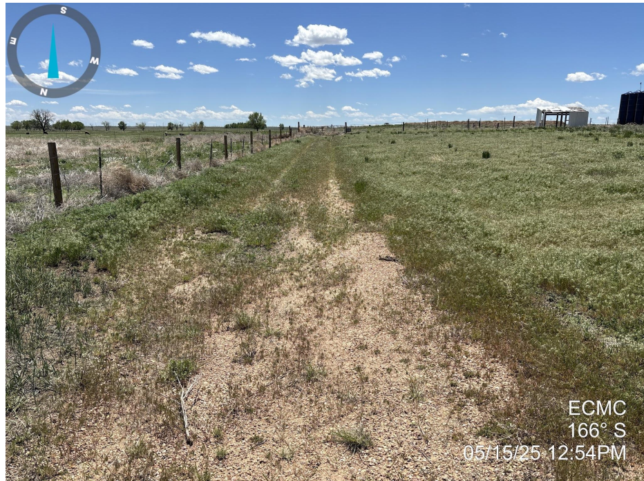
Photo 2. Photo taken from the access road, facing South. Photo illustrates that gravel remains across the access road and vegetation establishment does not meet Rule 1004 standards.
