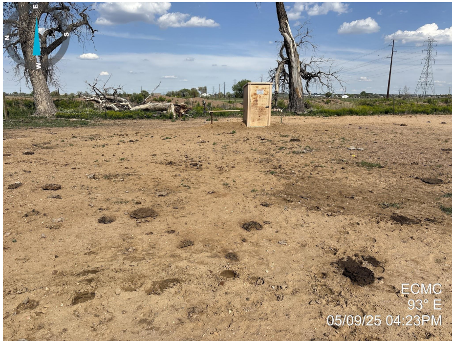
Photo 3. Photo taken from the tank battery location, facing East. Photo illustrates that final reclamation activities do not appear to have taken place and the meter house remains on location.
