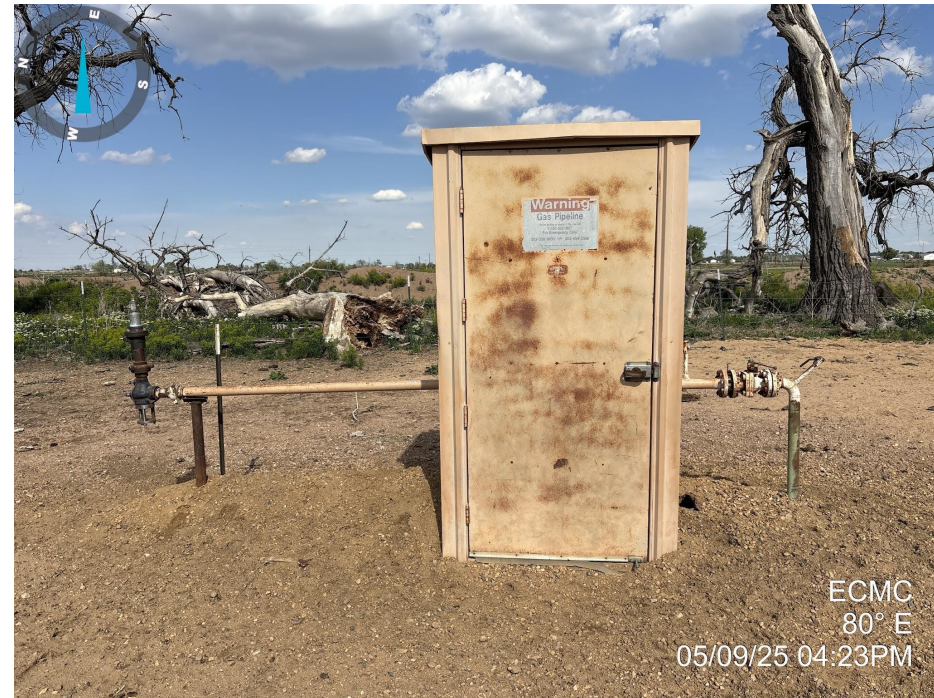
Photo 4. Photo taken from the well location, facing East. Photo illustrates the meter house which remains on site and is no longer in use.
