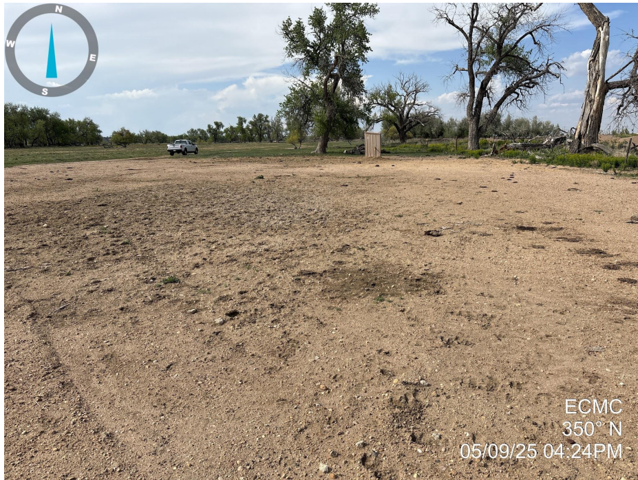
Photo 1. Photo taken from the tank battery location, facing North. Photo illustrates that final reclamation activities have not taken place and gravel and bare ground remains at the location.
