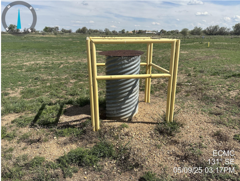
Photo 9. Photo taken of the tank battery location, facing Southeast. Photo illustrates that a buried valve set for midstream equipment remains on location.
