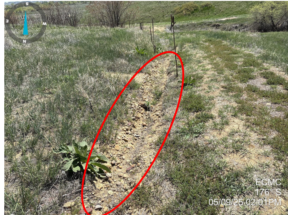
Photo 6. Photo taken of the access road, facing South. Photo illustrates that erosion is present along the side of the road (highlighted in red).
