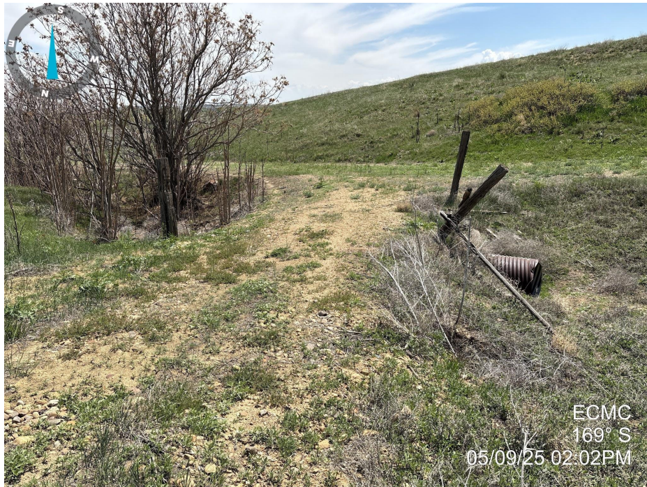
Photo 7. Photo taken of the access road, facing South. Photo illustrates that the access road has not been reclaimed and culverts remain along the road.
