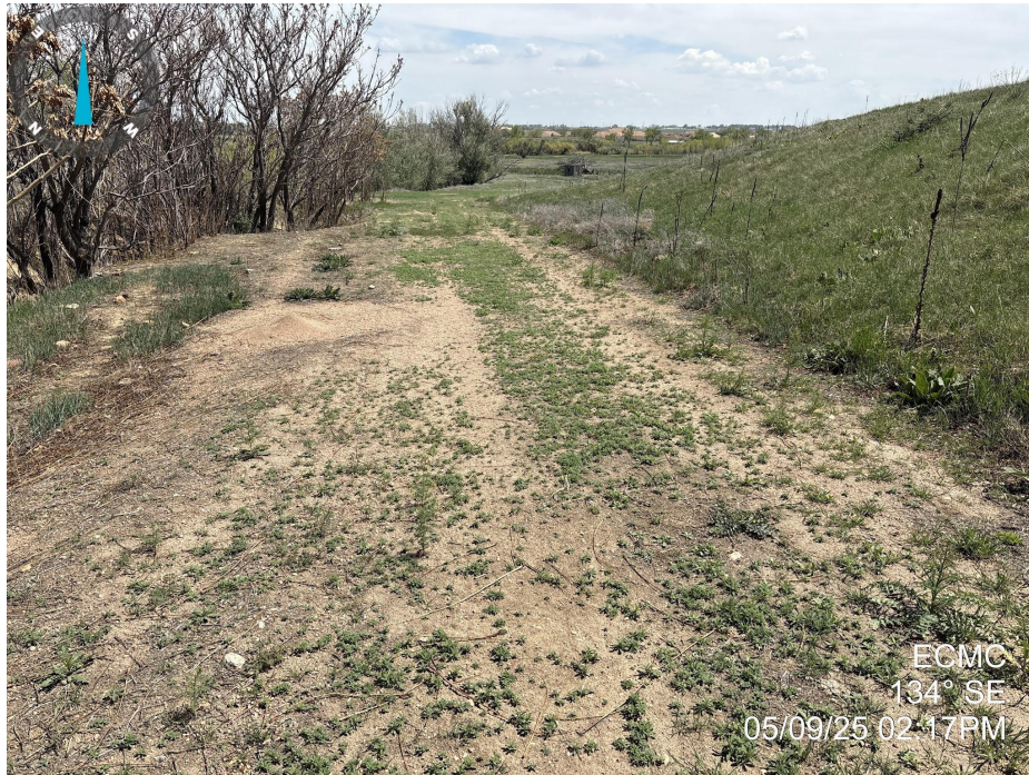
Photo 5. Photo taken from the access road, facing Southeast towards the location. Photo illustrates that the access road has not been reclaimed. Gravel remains on the road and weedy annual vegetation dominates the location.
