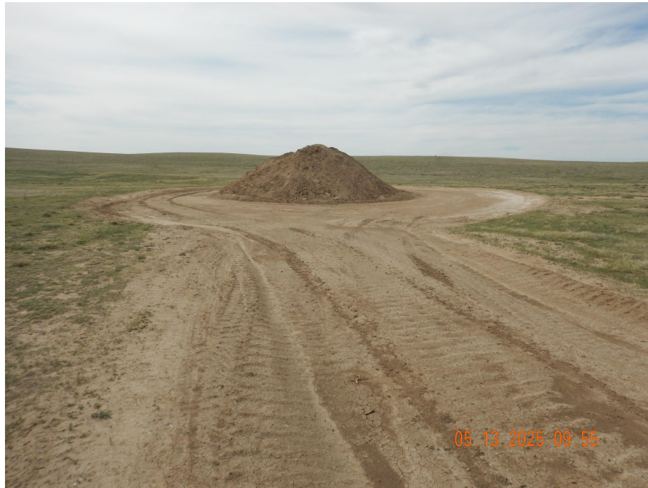
Photo 1. Photo taken from the northern location, facing South. Photo illustrates the Operator has stockpiled non-compliant topsoil and are waiting for soil lab results before hauling off the material.
