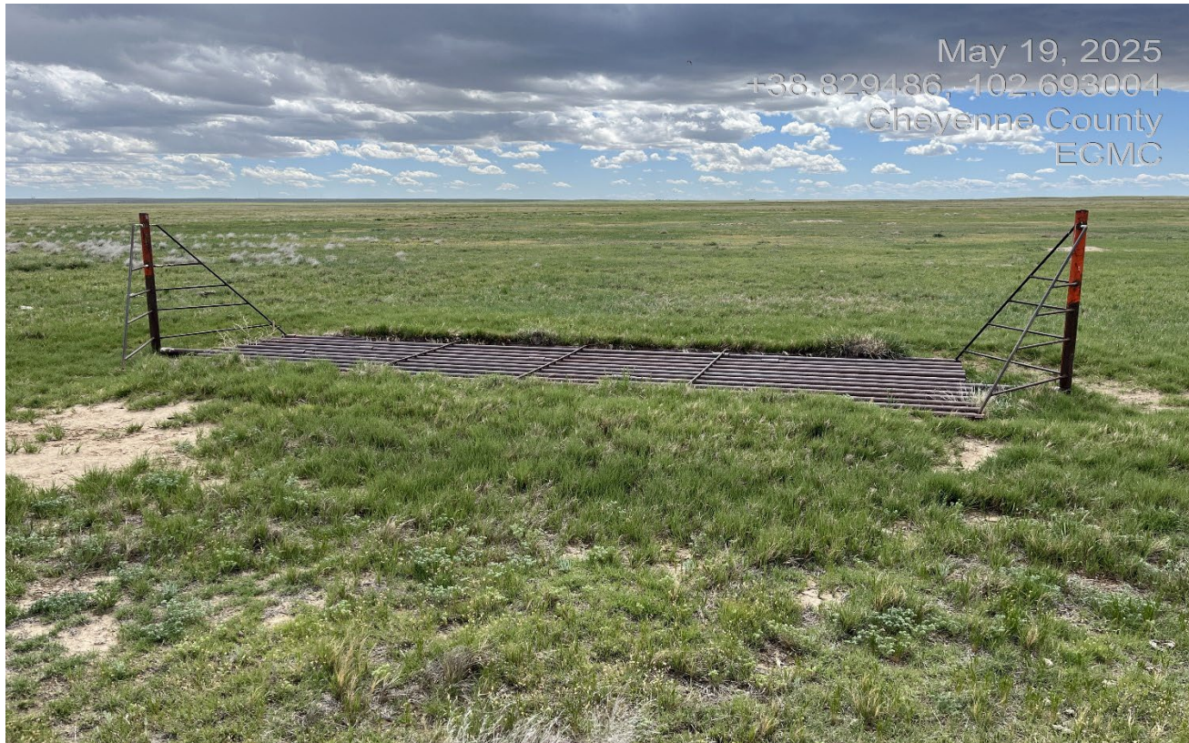
Photo 2. Facing southeast at the location. The cattleguard has not been removed from the location. The perimeter fence was removed but not the cattleguard.
