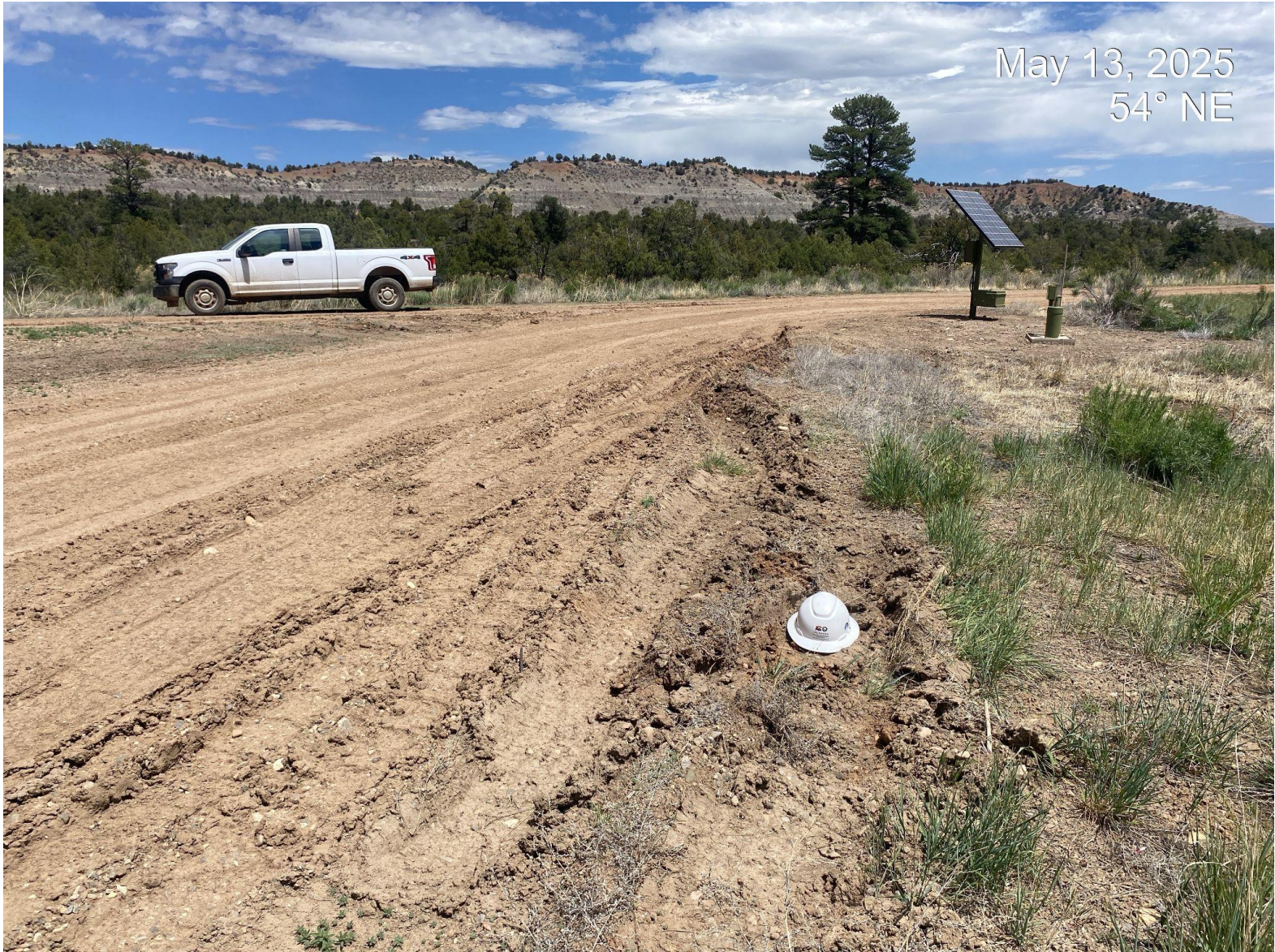
Photo 2. Rutting occurring at well pad access point.
