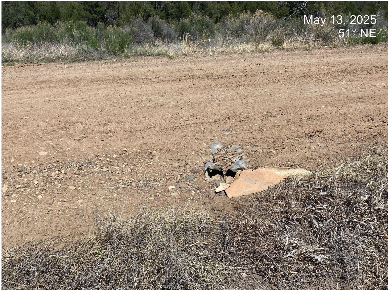
Photo 4. Damaged culvert at location access point.
