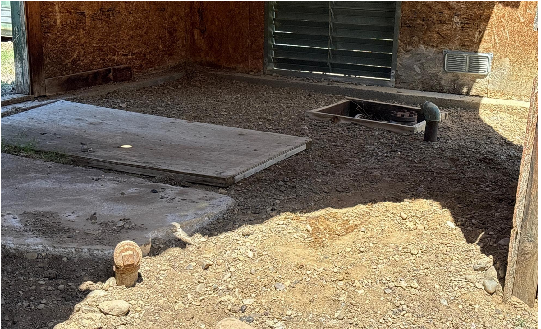
PHOTO 7: UNUSED EQUIPEMENT ( UNUSED RISERS NOT MARKED OR LABELED INSIDE UNUSED SHED). MARK OR REMOVE UNUSED AND OR UNNESSESARY RISERS PER RULE 606. CA DATE 6/14/2025.
