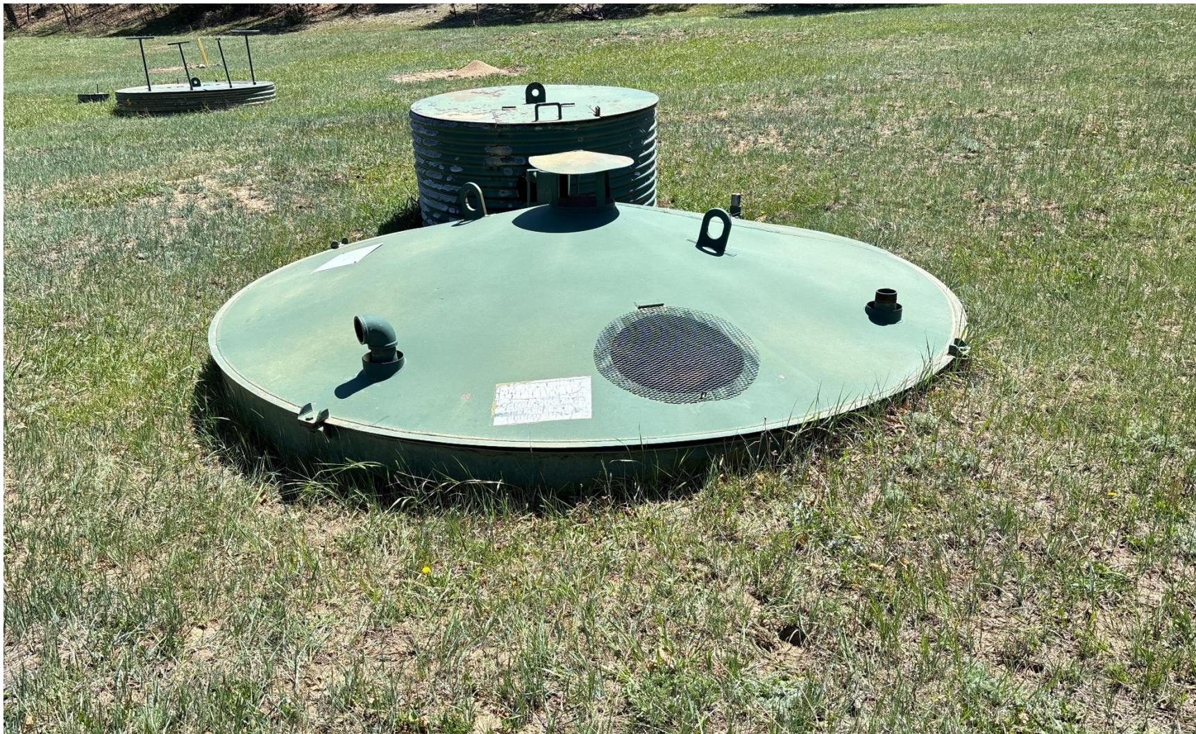
PHOTO 4: PRODUCED WATER TANK BATTERY. NFPA, CAPACITY AND CONTENTS NOT LABELED ON TANK. Install sign to comply with Rule 605.h. CA DATE 5/19/2025.
