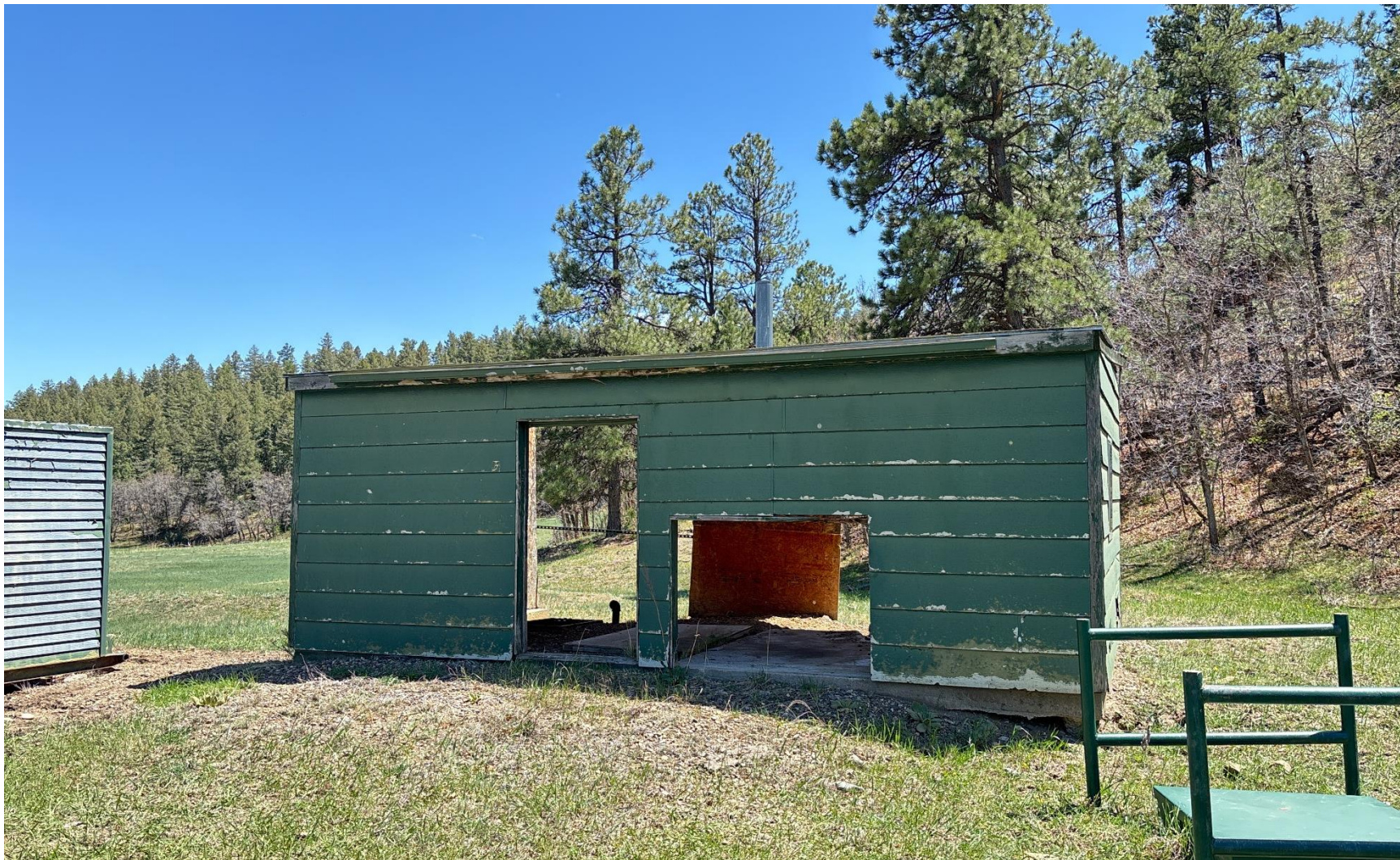
PHOTO 6: UNUSED EQUIPMENT (SHED DOES NOT APPEAR TO BE IN USE OR USEFUL TO THE OPERATION OF THIS FACILITY, SHED IS DETERIORATING AND TRASH AND DEBREE FROM SHED IS ON AND AROUND LOCATION). REMOVE UNUSED EQUIPMENT PER RULE 606. CA DATE 6/14/2025.
