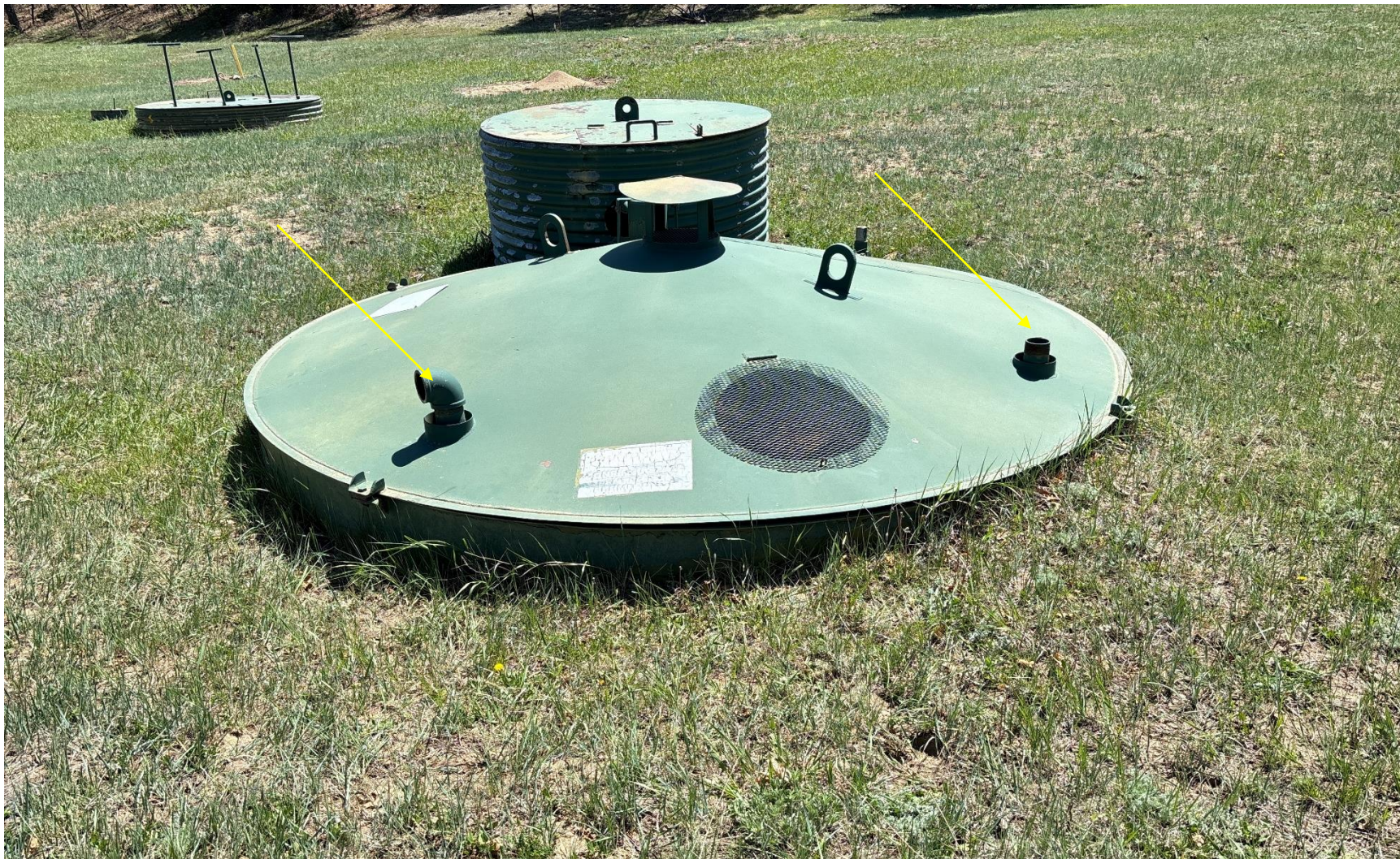
PHOTO 5: BIRD PROTECTORES MISSING OR NOT INSTALLED ON TWO PIPES IN TOP OF TANK. INSTALL BIRD PROTECTORS. CA DATE 5/19/2025.
