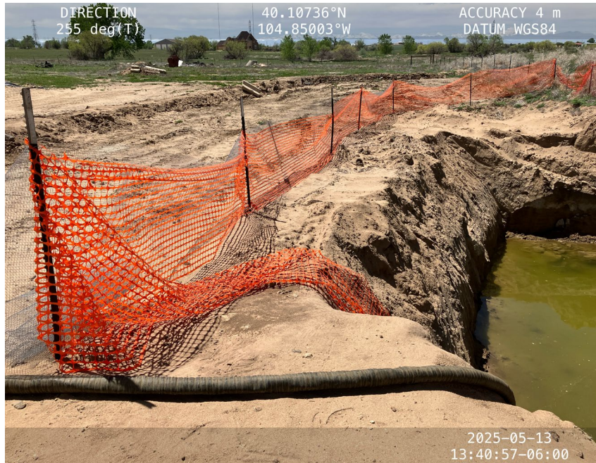
Excavation fencing has fallen
