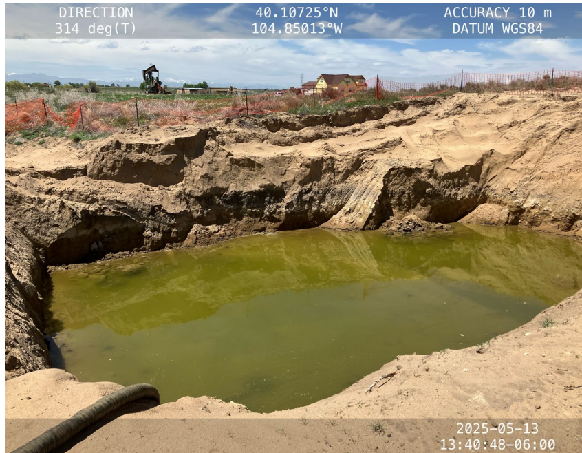
Excavation with Groundwater observed
