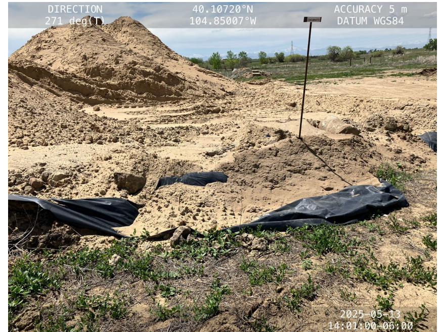
Contaminated soil is overflowing onto the ground past the liner
