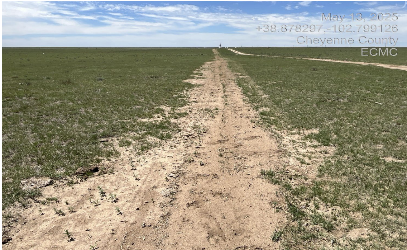
Photo 9. There has been new disturbance from a buried electric line to service the new electric motor at the pumpjack. The disturbed area will need to be reclaimed. Previous corrective action was not completed.
