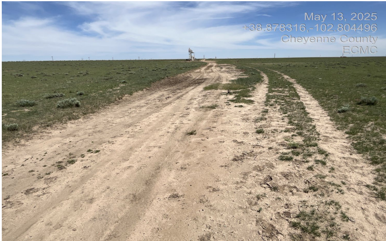
Photo 2. Facing east along the access road. Another area where vehicles caused unnecessary disturbance driving outside of the access road due to stormwater pooling on the road. BMP's have not been installed to stabilize the road and the disturbance has not been reclaimed.
