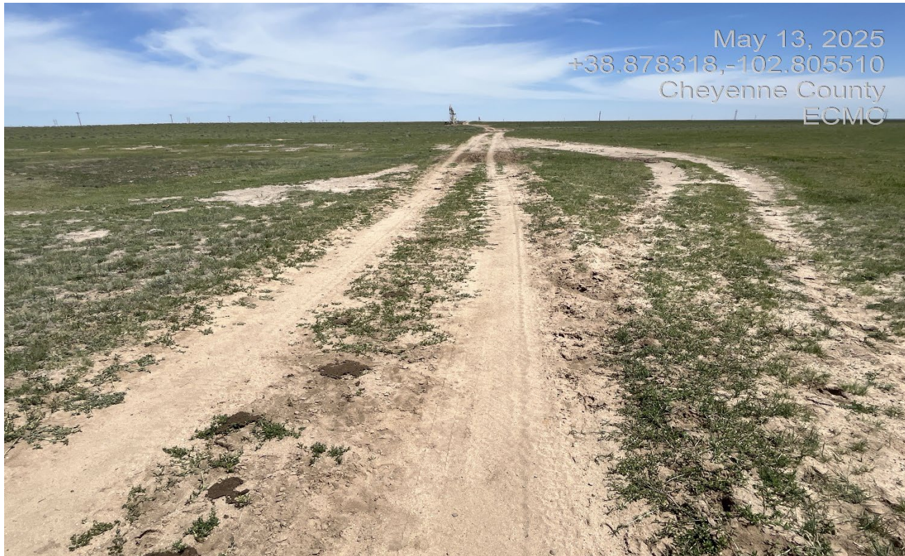
Photo 1. Facing east along the access road. Vehicles caused unnecessary disturbance driving outside of the access road due to stormwater pooling on the road. BMP's have not been installed to stabilize the road and the disturbance has not been reclaimed.
