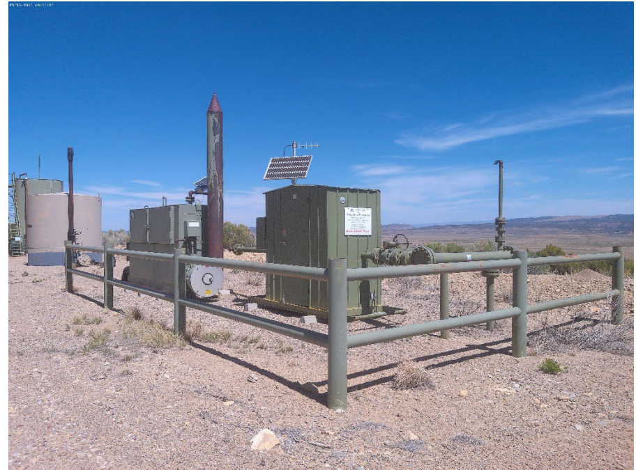
Separator and Meter housing
