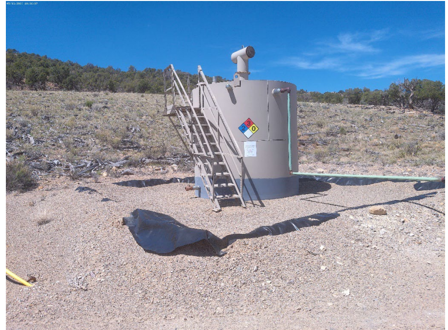
Tank battery Berms inadequate
