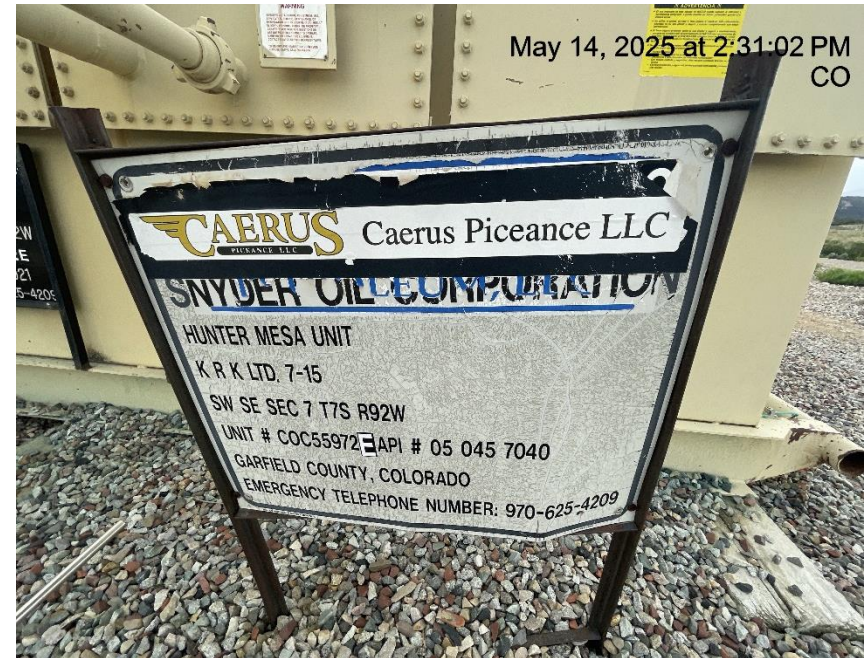
Photo # 1541 Emergency phone # on wellhead sign incorrect/# is disconnected & not in service
