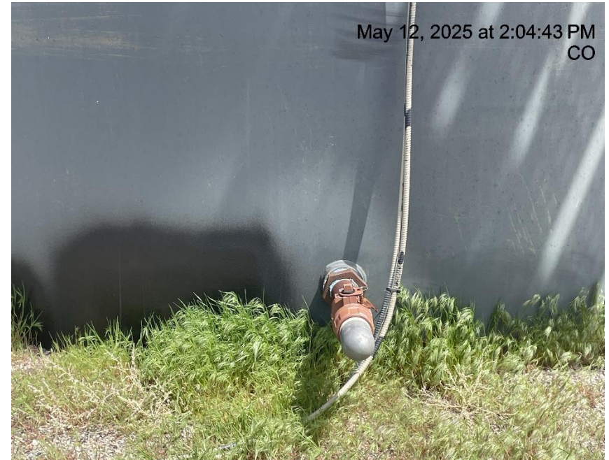
Photo # 324 Weeds in secondary containment
