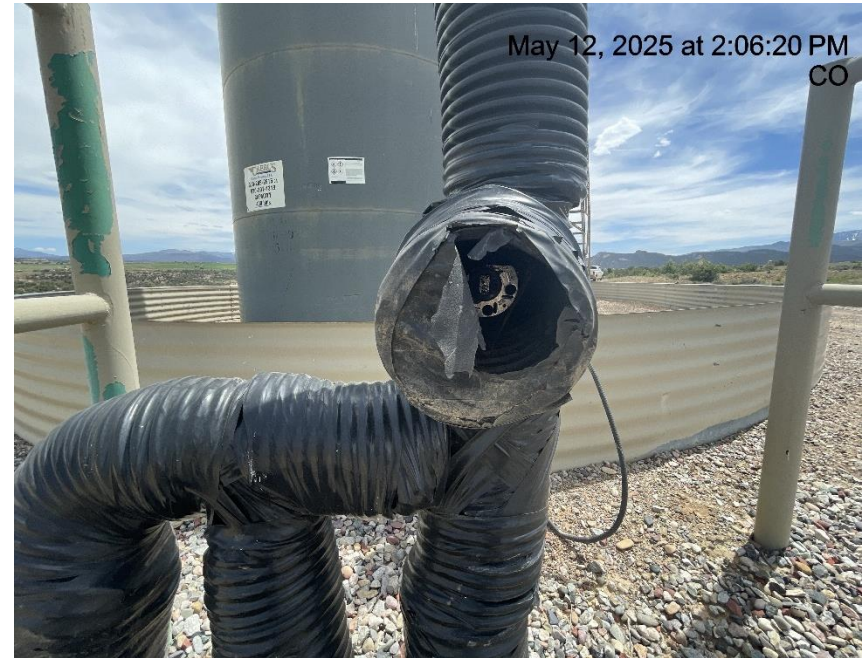
Photo # 322 Flowline heating insulation open ended/wildlife hazard/available for entry by wildlife
