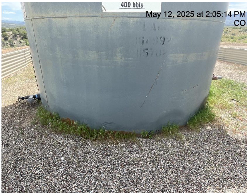
Photo # 323 Weeds in secondary containment
