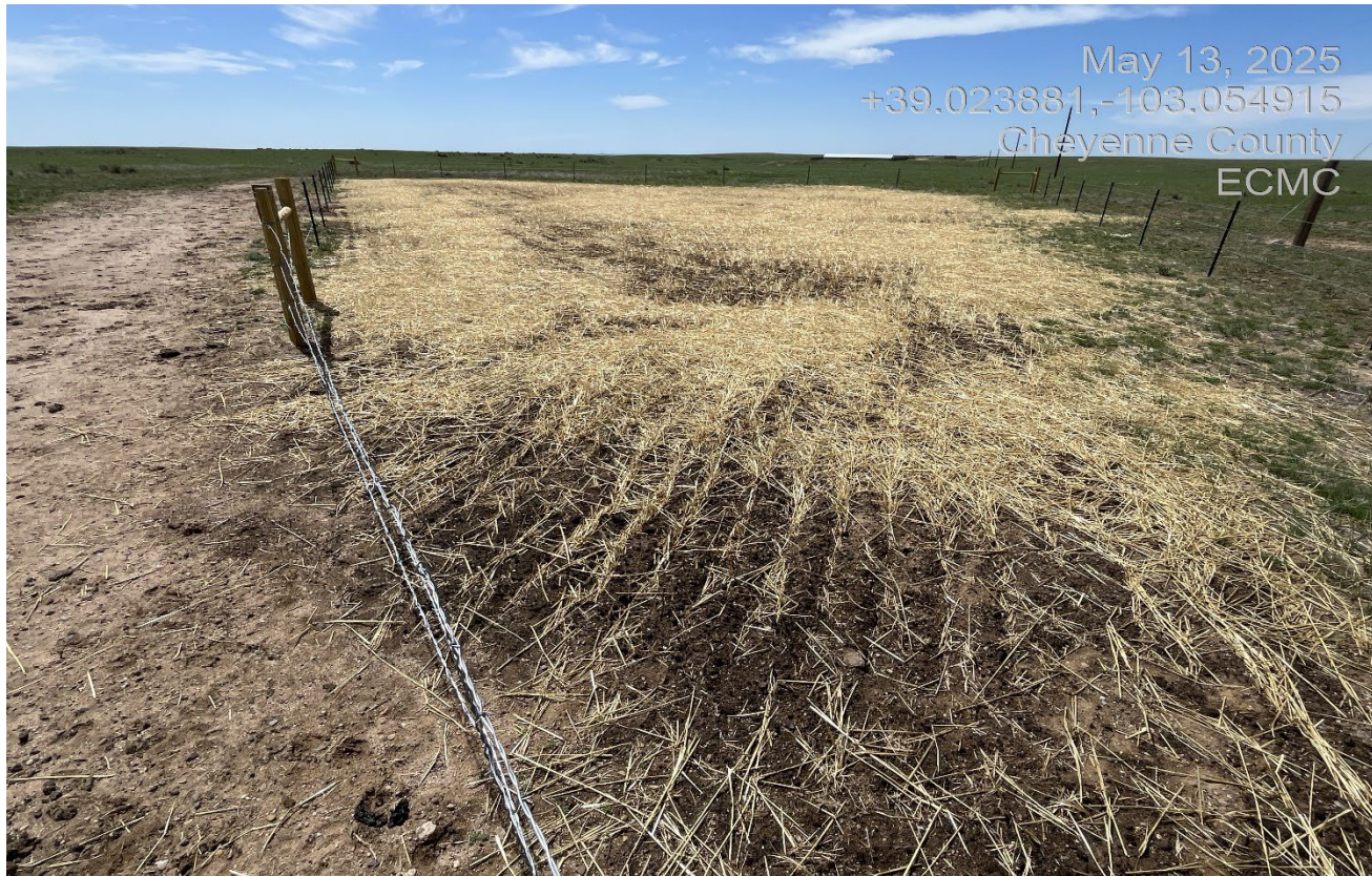
Photo 3. Facing south at the location. The soils have been decompacted and seeded. There was manure and straw mulch applied to disturbed areas.
