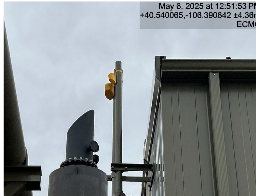
Rain caps not installed properly
