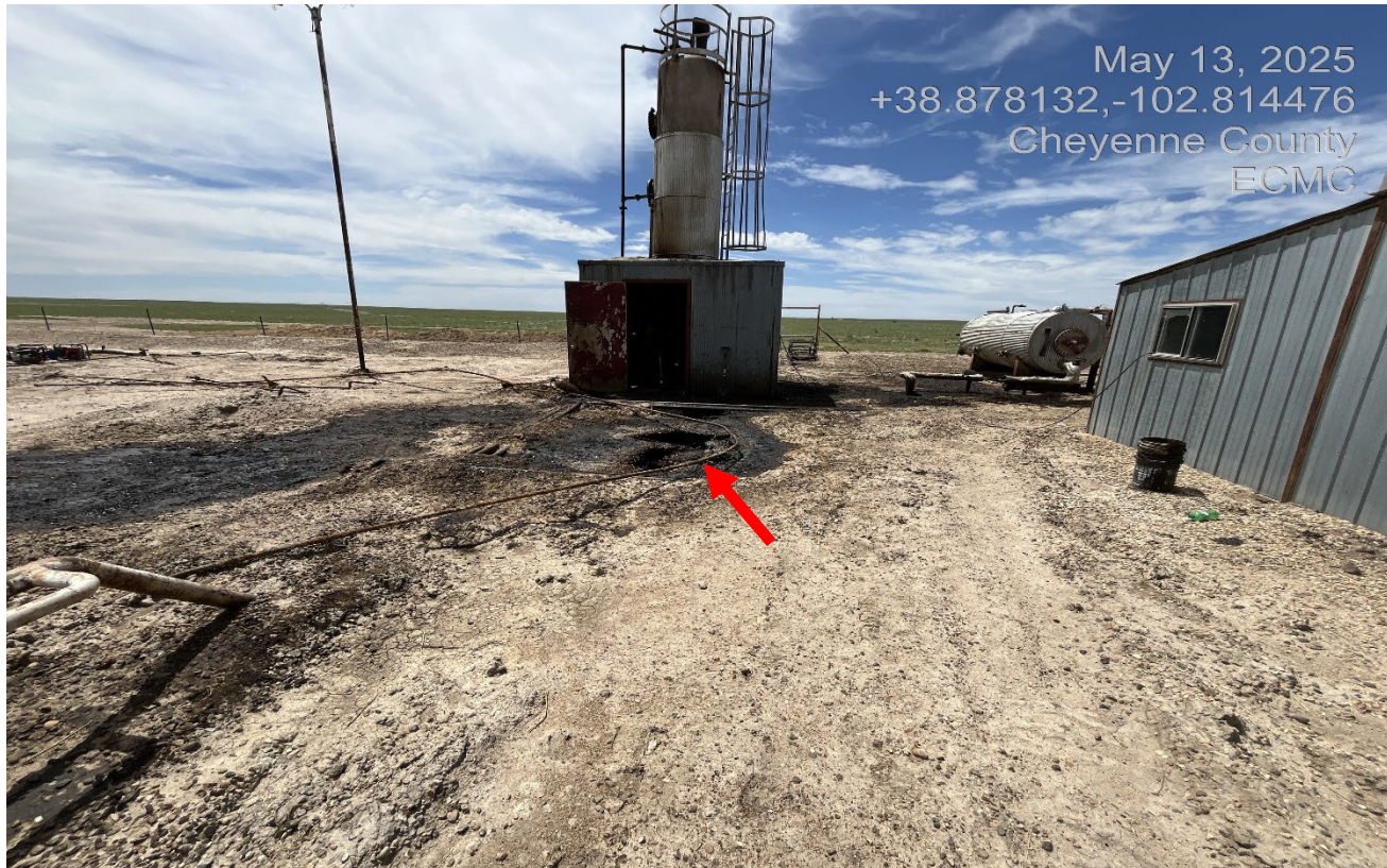
Photo 12. There is puddled oil free fluids shown at red arrow that needs immediate clean up.
