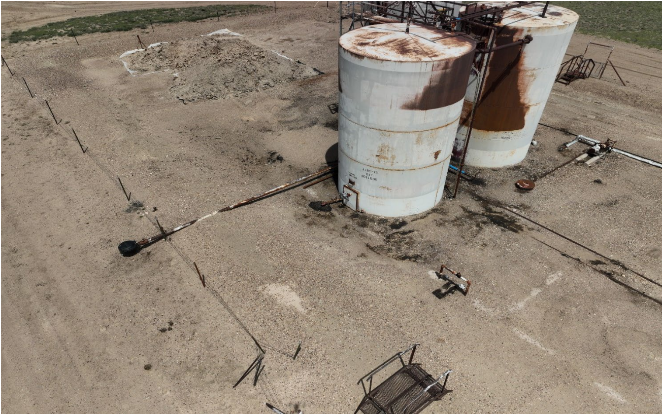
Photo 5. Drone aerial photo facing down toward the north side of the tank battery. Oil stained soils still remain around the tanks and have not been cleaned up.
