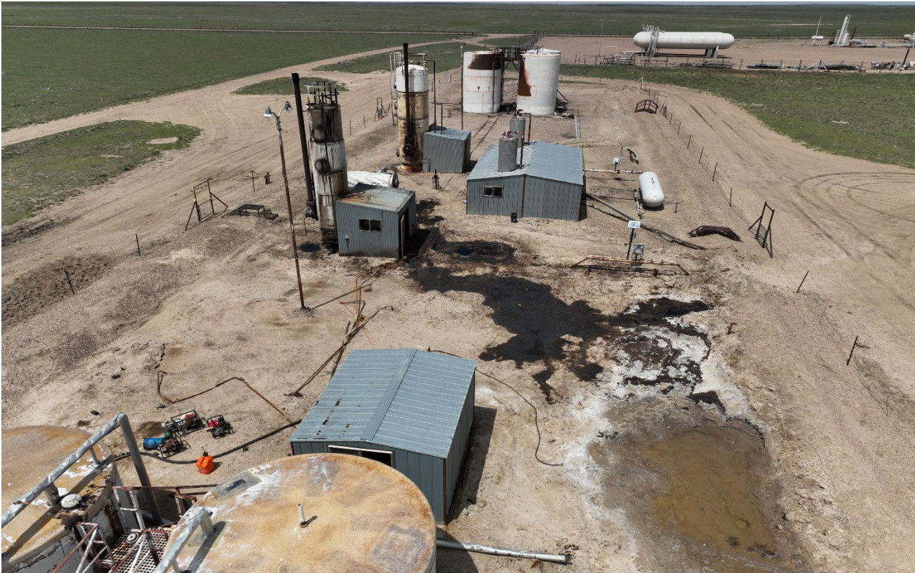
Photo 3. Drone aerial photo facing northwest toward the tank battery facility. There is a new spill that has recently occurred in addition to previous spills at this same area and at the same equipment.
