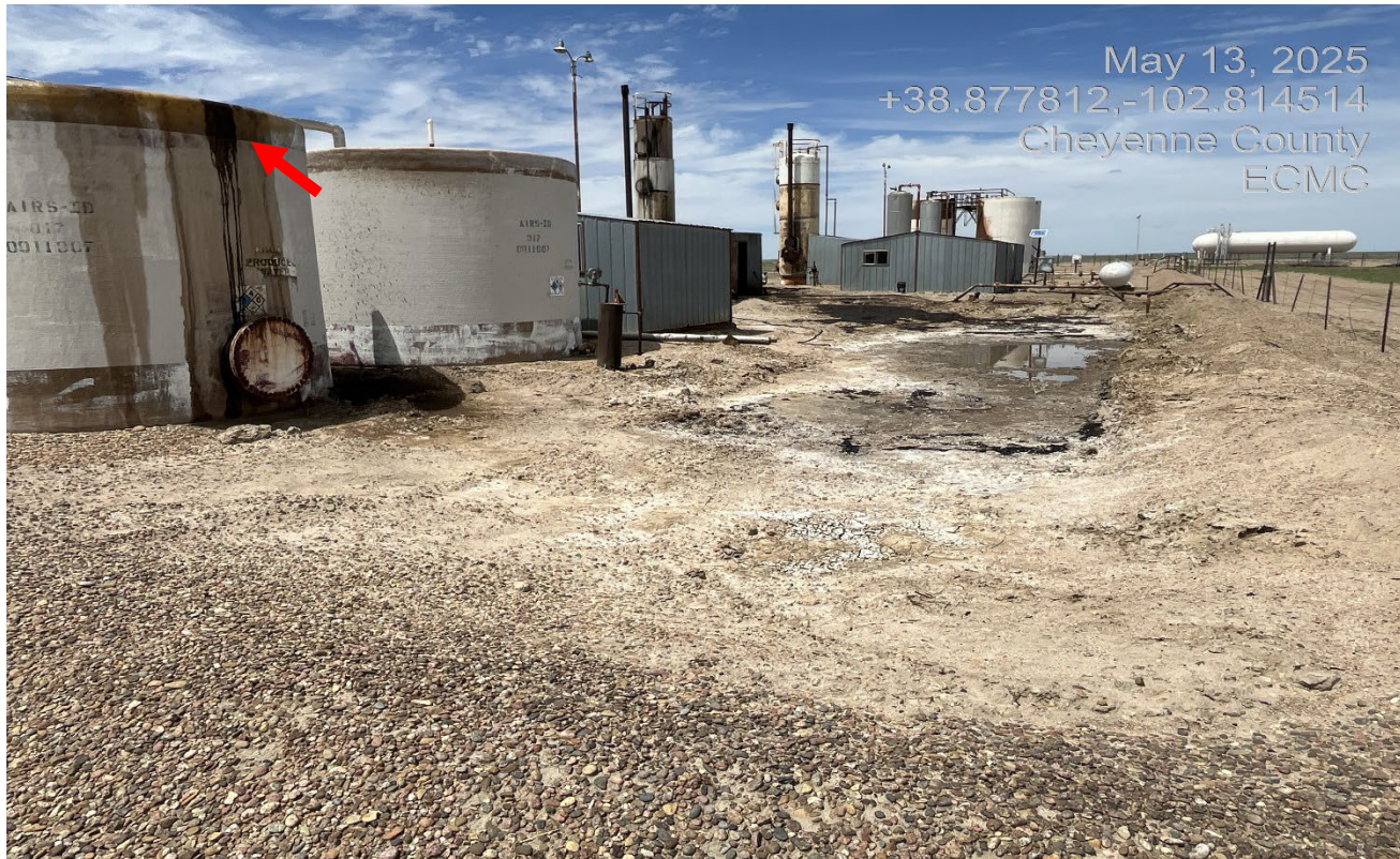
Photo 10. Southeast corner of the location facing northwest toward the tank battery facility. There are signs of a leak at the top of the fiberglass tank shown at red arrow.
