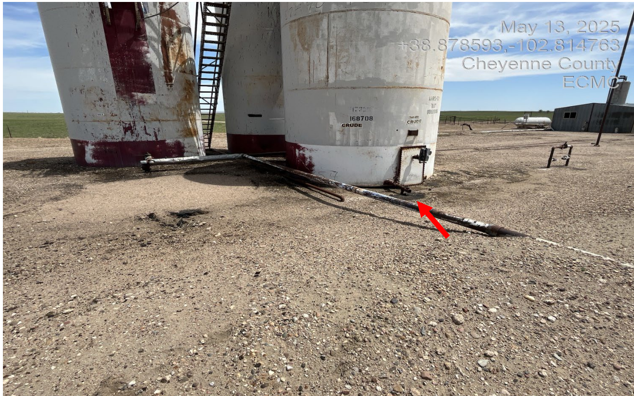
Photo 8. Facing southeast toward the tank battery. The oil stained waste remains around the tanks. Some of the tanks were removed since the previous inspection.
