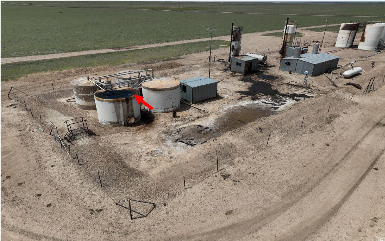
Photo 2. Drone aerial photo facing northwest toward the tank battery. There is oily liquid shown on top of the tank at red arrow which need to be cleaned up and properly disposed. Previous corrective action was not completed.
