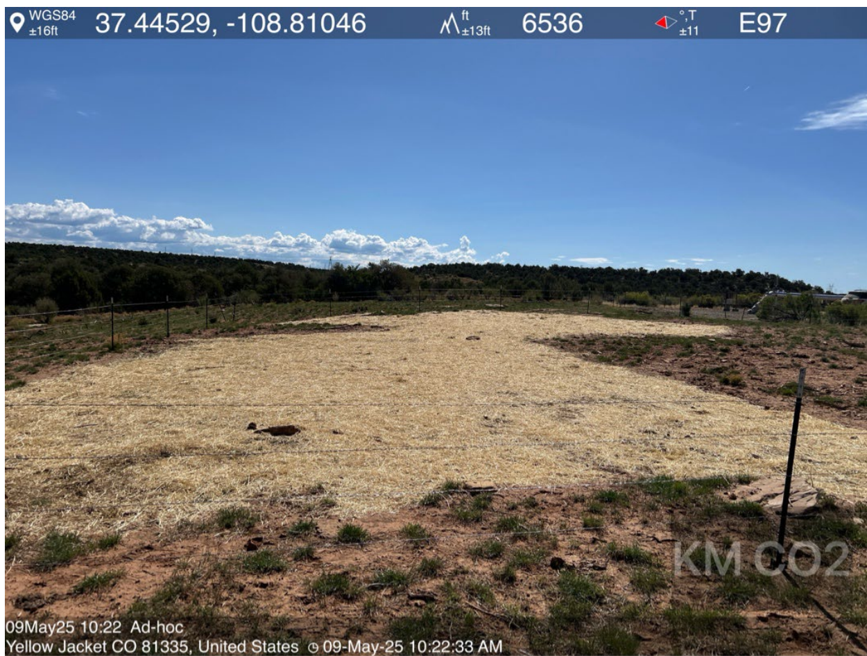
Photo #4. View of the YB-2 well location, reseed, straw, fencing application.
