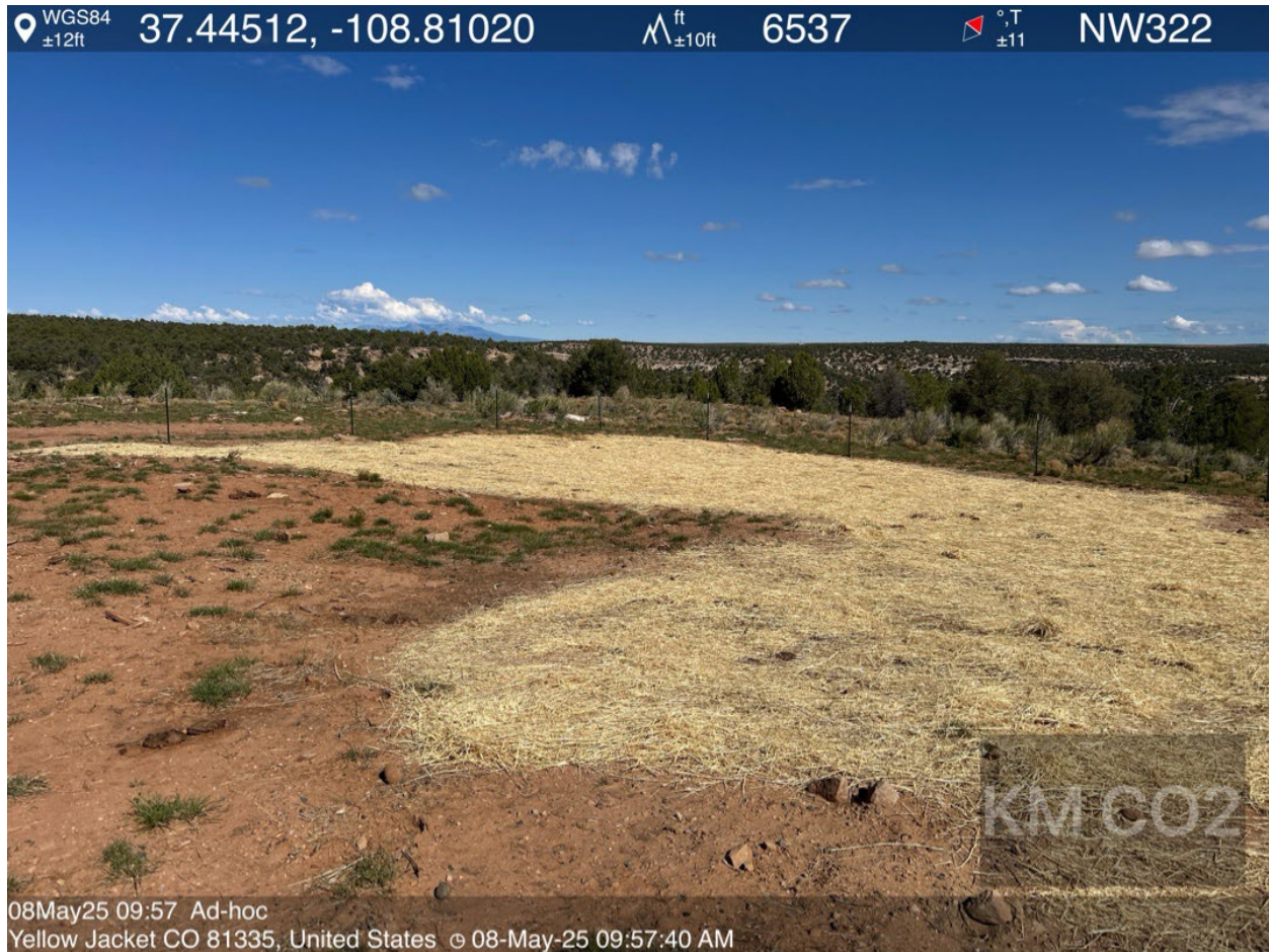
Photo #3. View of the YB-2 well location, reseed, straw, fencing application.
