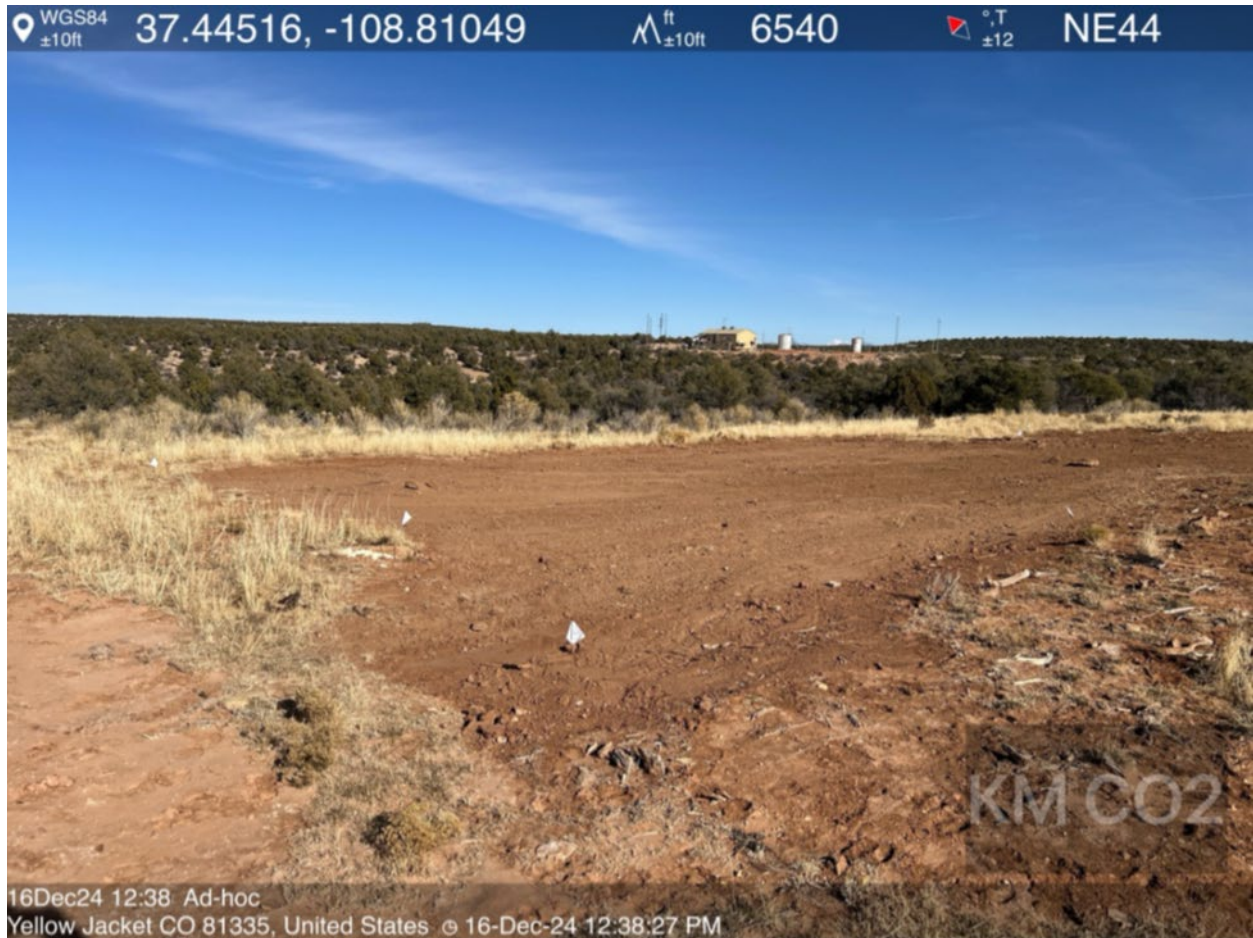
Photo #2. View of the YB-2 well location, topsoil application.
