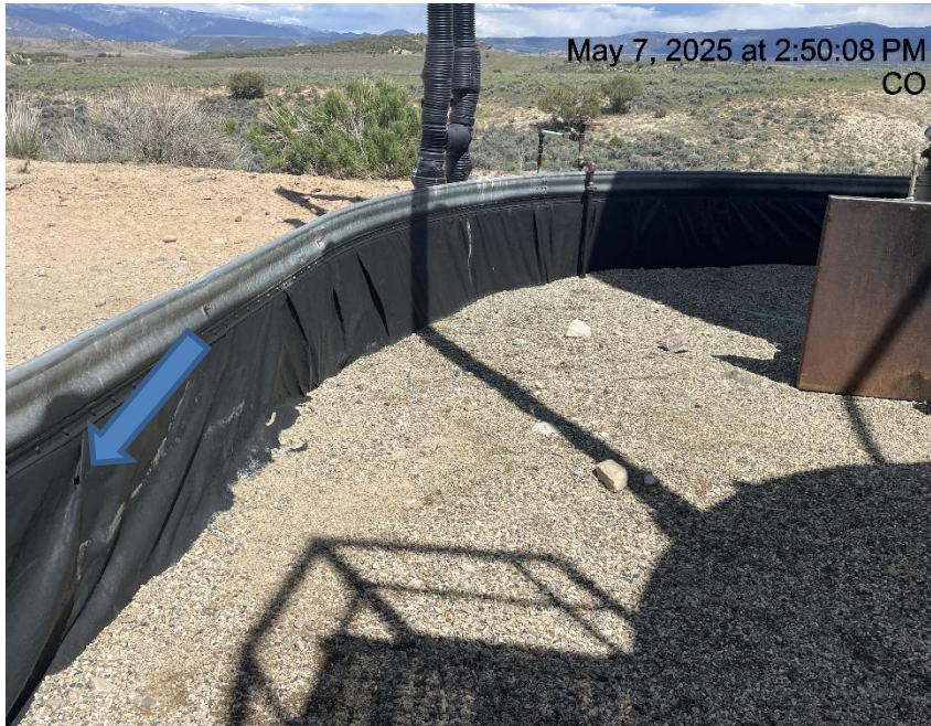
Photo # 9566 Hole in secondary containment liner/liner needs maintenance
