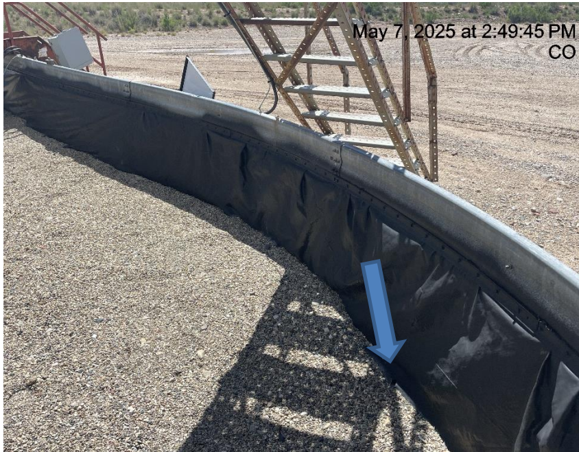
Photo # 9564 Hole in secondary containment liner/liner needs maintenance
