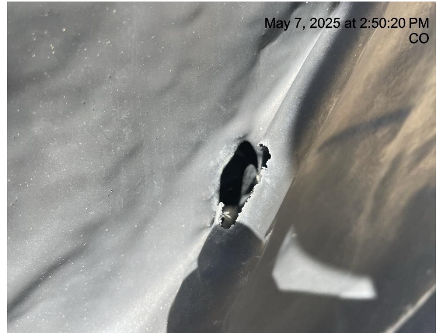
Photo # 9567 Hole in secondary containment liner/liner needs maintenance
