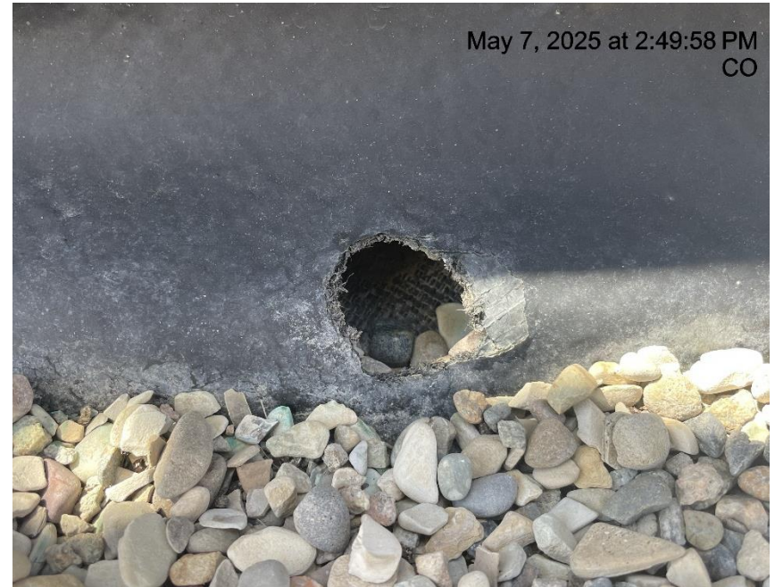
Photo # 9565 Hole in secondary containment liner/liner needs maintenance
