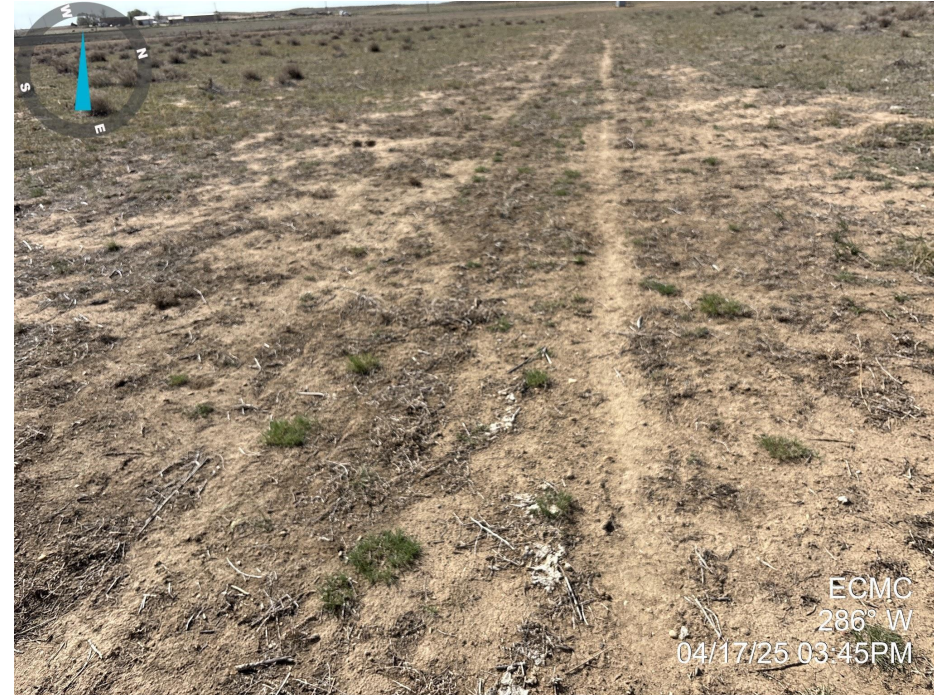
Photo 6. Photo taken from the access road, facing west, away from the well location. Photo illustrates that final reclamation activities have taken place, with evidence of drill rows, but vegetation establishment does not meet final reclamation standards.
