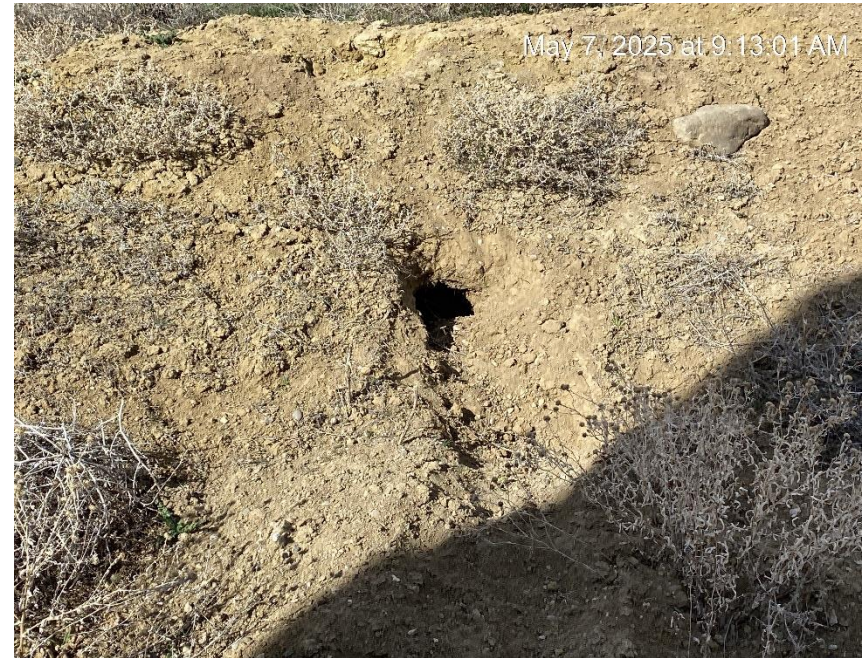
Tank berm burrow
